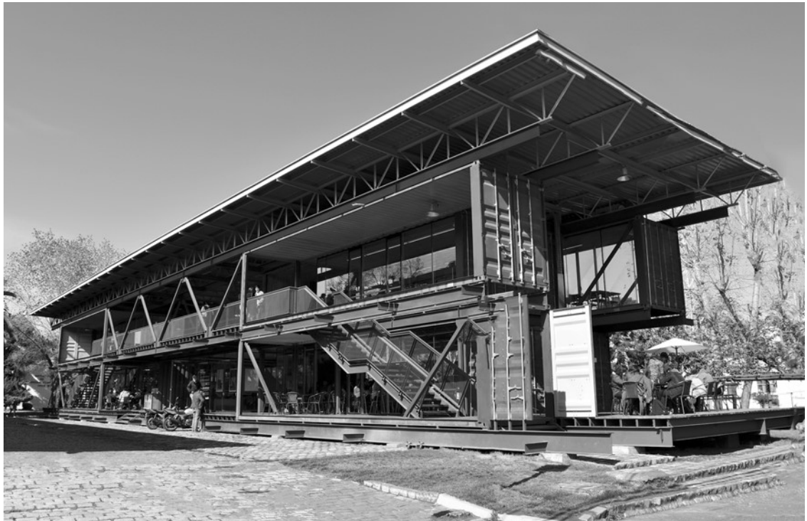
Two-story container-based structure used for classroom/meeting space. Courtesy of Modular Building Institute.
