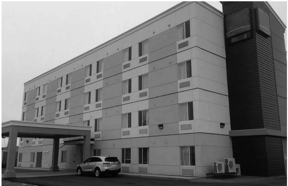
Four-story constructed utilizing shipping containers. Courtesy of the Modular Building Institute.
