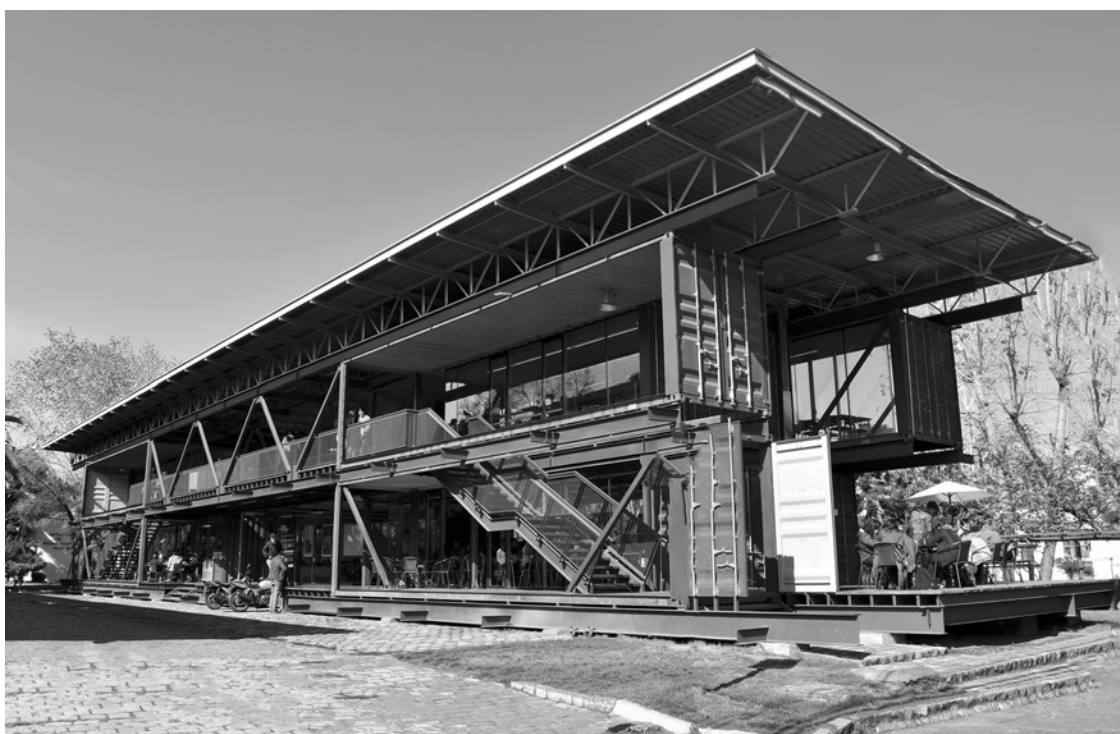
Two-story container-based structure used for classroom/meeting space. Courtesy of Modular Building Institute.
