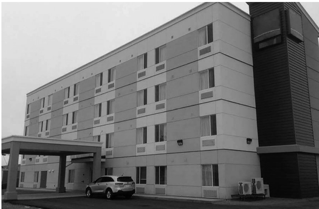
Four-story constructed utilizing shipping containers. Courtesy of the Modular Building Institute.
