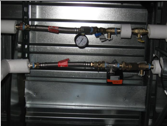
Piping Pressure Test Gauge on VAV Branch HW Piping
