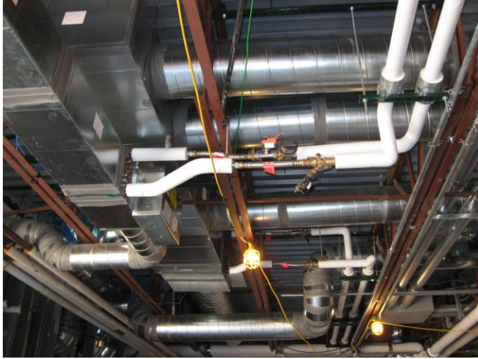
VAV-01 Installation
