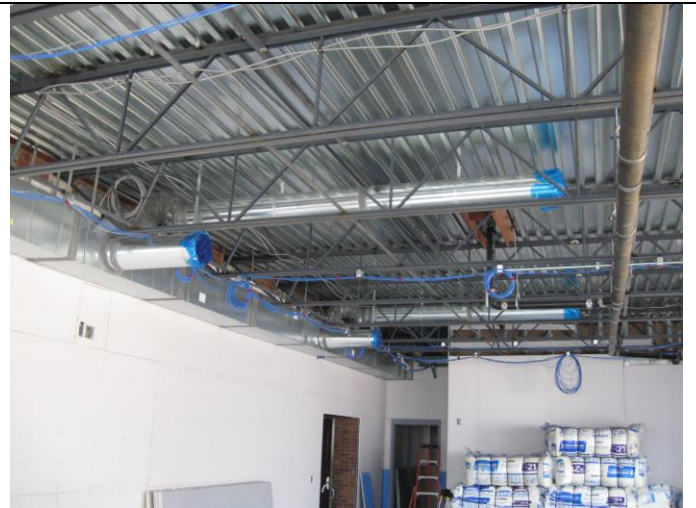
Music Classroom: Main and Branch Ductwork Installed
