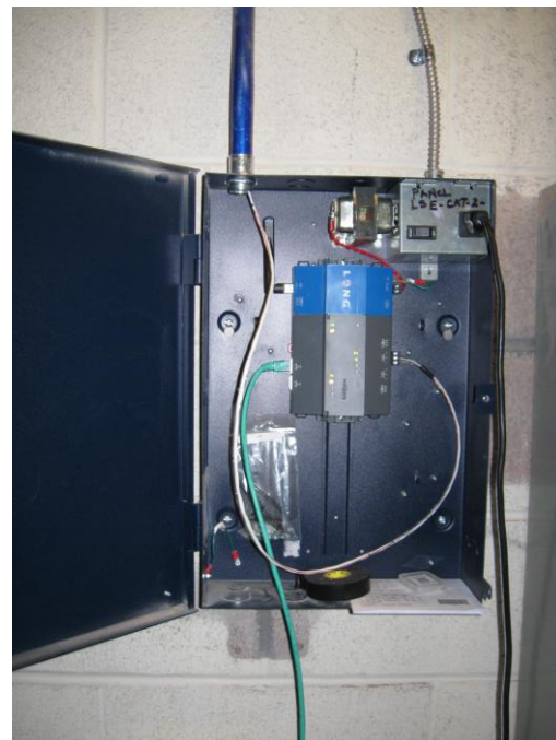
New JACE Controller with Niagara
