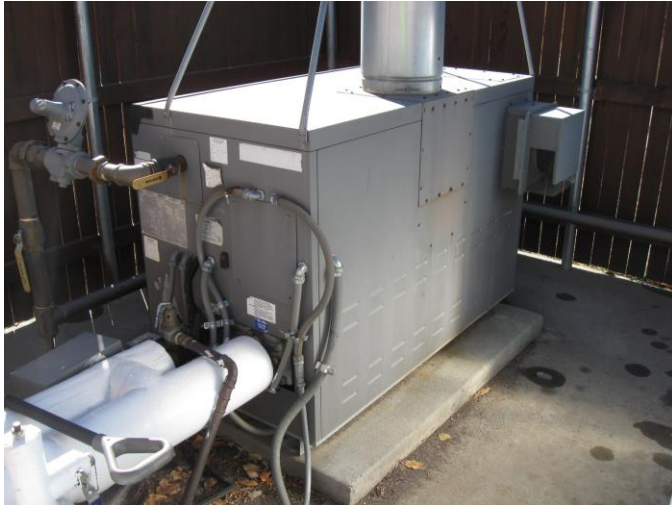
Existing Snowmelt Boiler – SB-3 serving New Snowmelt Area
