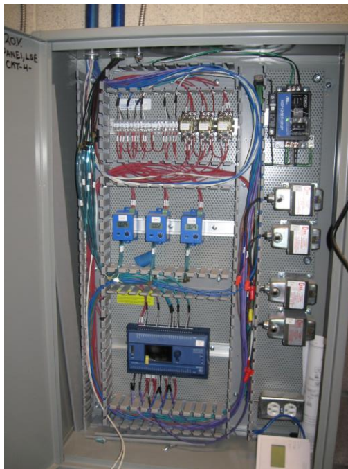
New BAS Control Panel with AHU Controller
