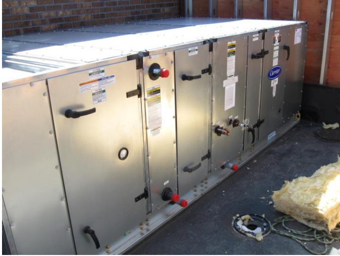
AHU-2 Installation
