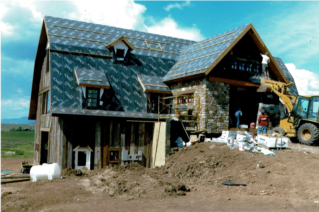
PHOTO SHOWS BUILDING WRAP AND ROOF BITUTHANE INSTALLATION WHICH MEETS 2015 I.R.C. REQUIREMENTS.
