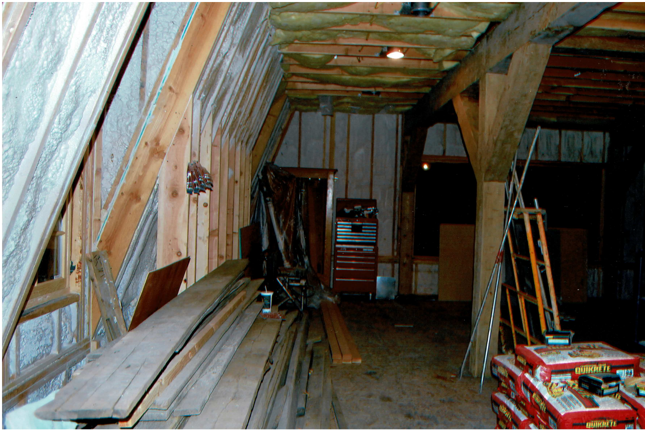
PHOTO SHOWS SPRAY FOAM INSULATION FULL DEPTH IN WALL CAVITY. INSULATION MEETS 2015 I.E.C.C. VALUES.
