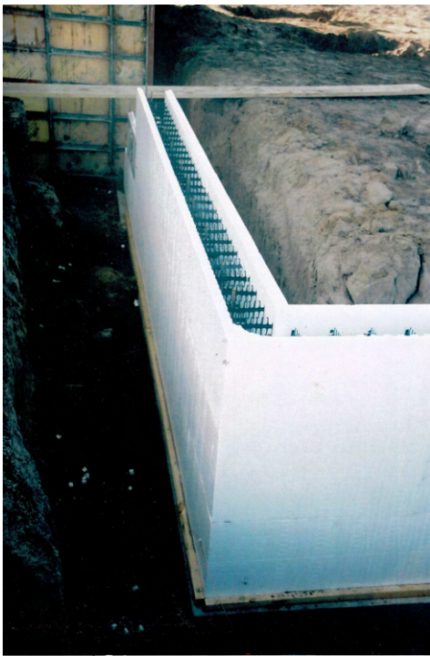
PHOTO SHOWS FOUNDATION INSTALLATION WITH INSULATED CONCRETE FOUNDATION BLOCKS MEETING 2015 I.E.C.C.
