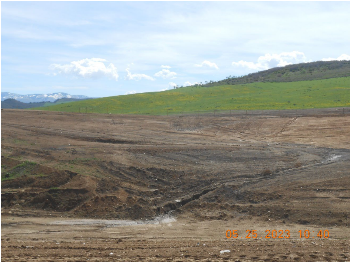
Photo 19: Excavation area for Module (MOD) 8 expansion area (note channel dug to convey runoff from area above and seepage area)
