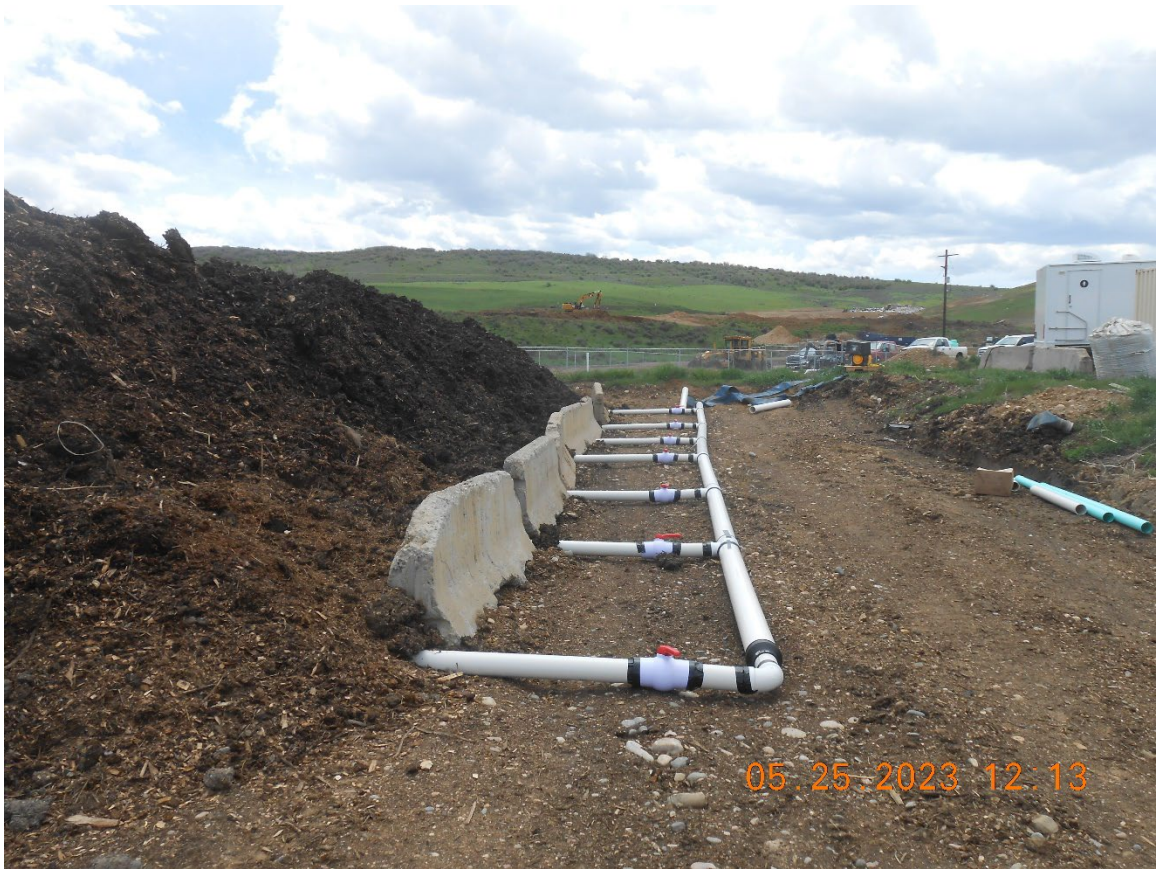
Photo 31: Aeration system along western side of compost work pad (blowers did not appear to be connected at time of inspection)
