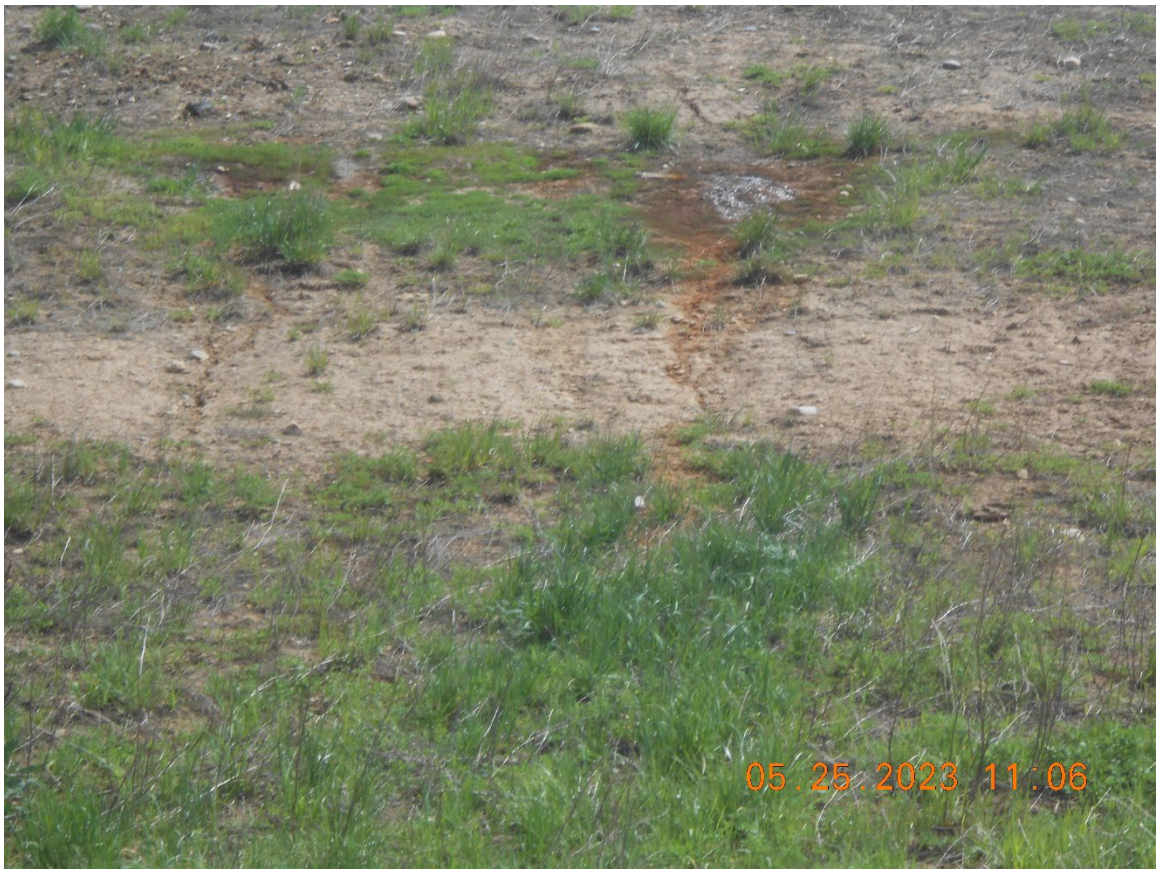
Photo 21: Small seep on side slope of landfill (western slope)
