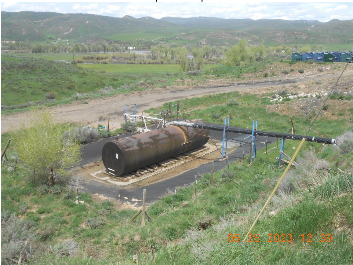
Photo 38: Leachate holding tank and surrounding containment
