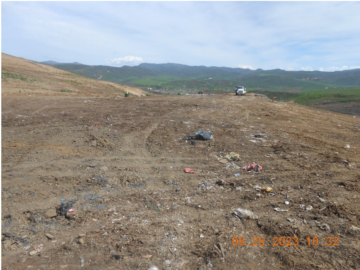
Photo 15: Insufficient cover noted south of the working face area
