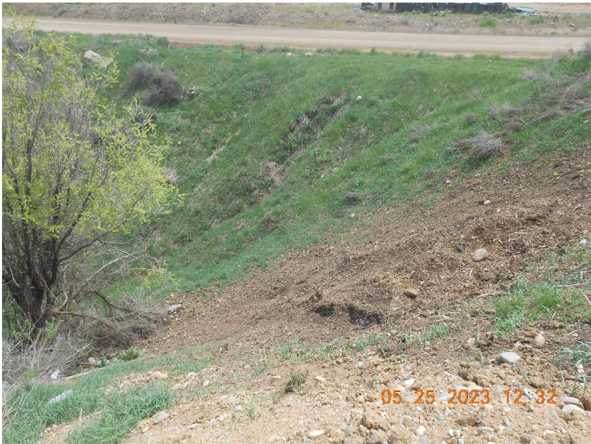
Photo 35: View looking east / northeast showing compost material had been pushed down the slope on eastern side of compost area
