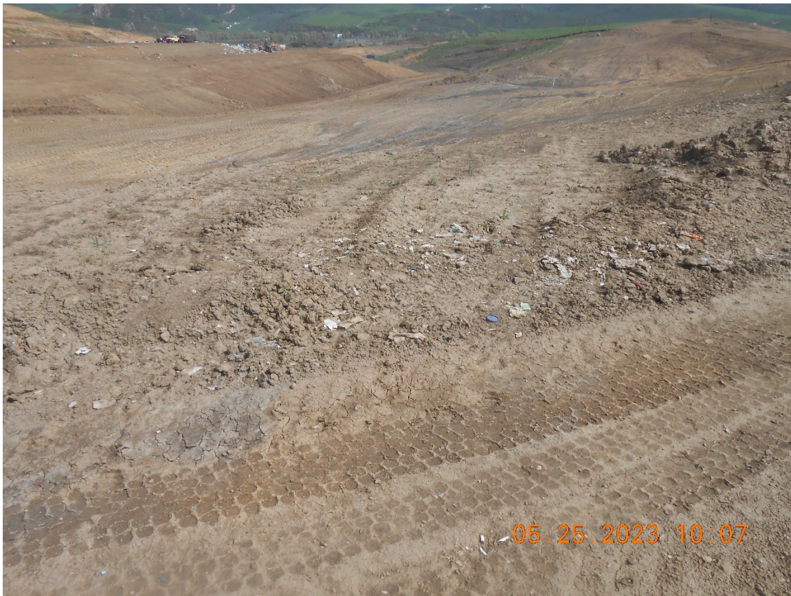
Photo 13: Area to the south of the MOD 8 excavation area (note no berm was present in this area to prevent run-on into the MOD 8 excavation area)
