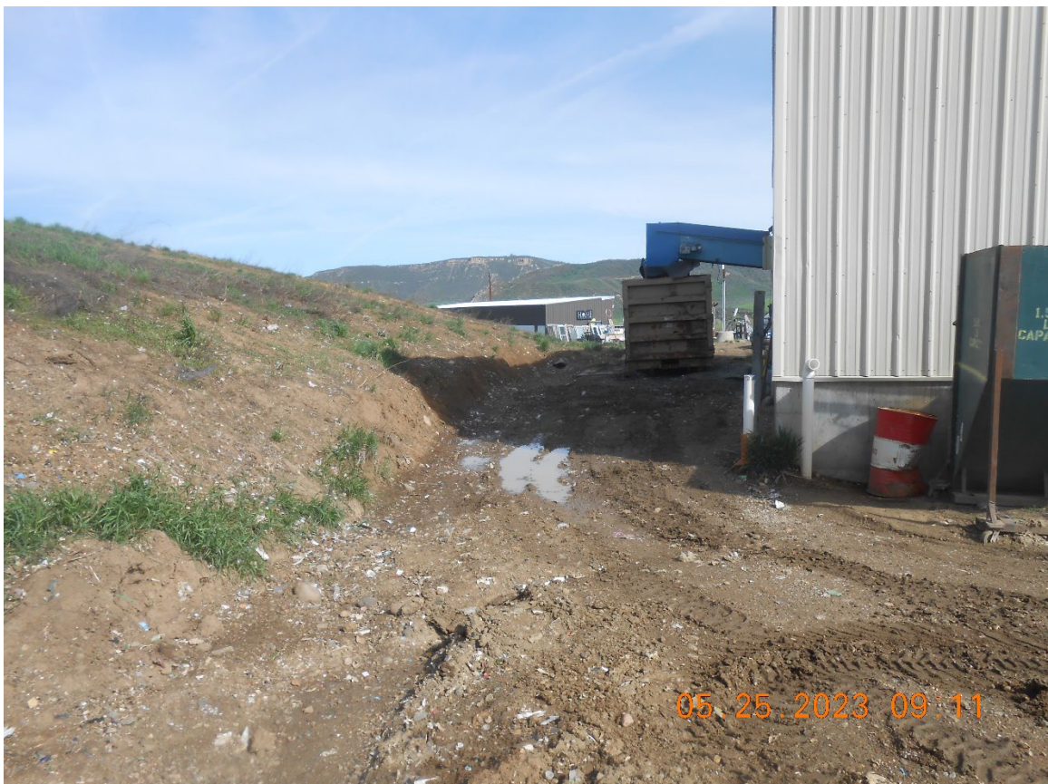
Photo 6: Area west of MRF (note debris on ground and lack of drainage (this drainage is continuous from drainage channel shown in Photo 5))
