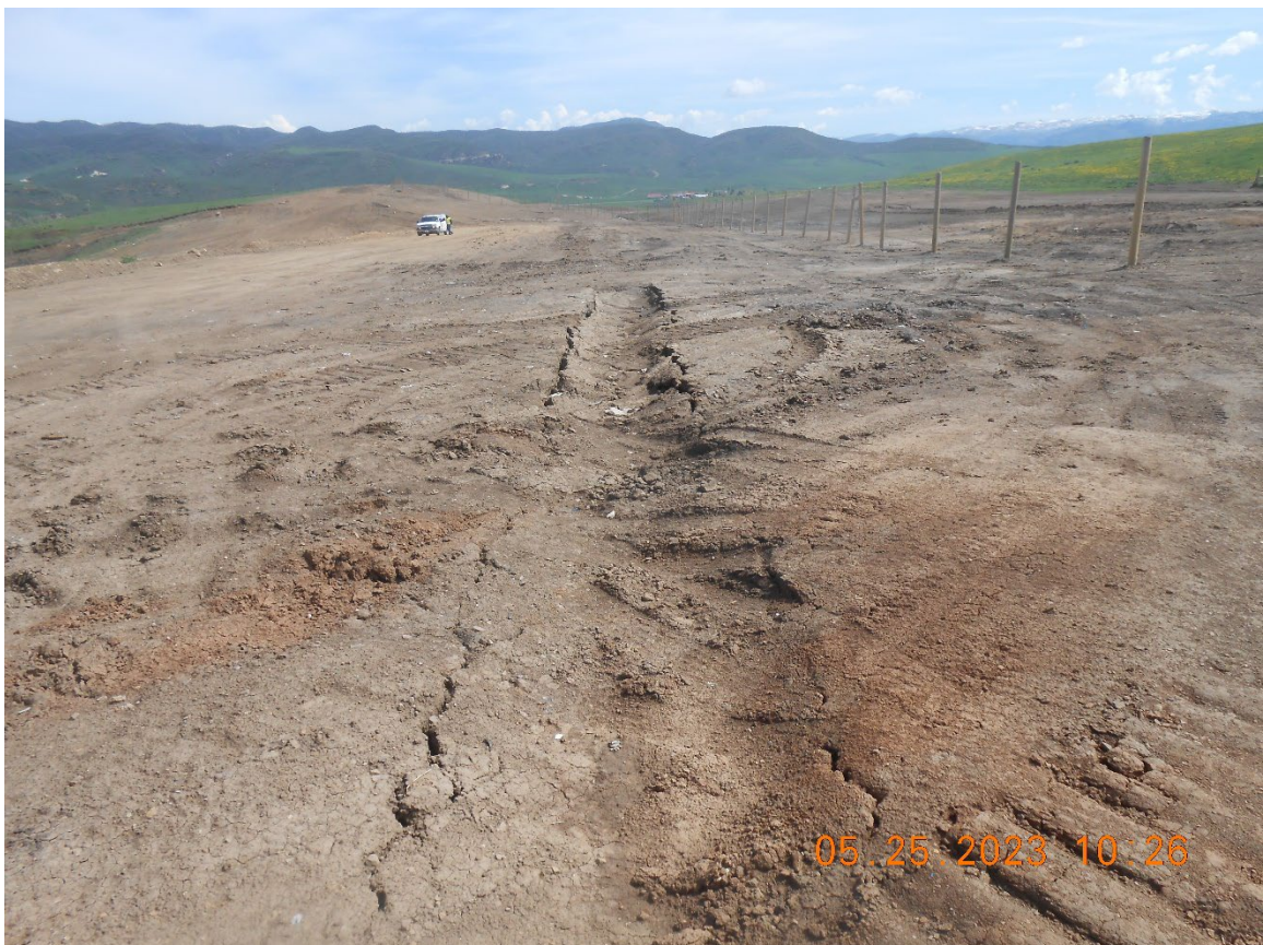
Photo 12: Collapsing ground surface presumably due to saturated conditions
