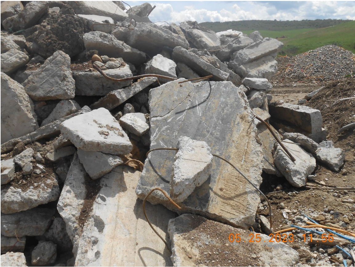
Photo 23: Concrete staged for recycling (note presence of sealant on concrete)
