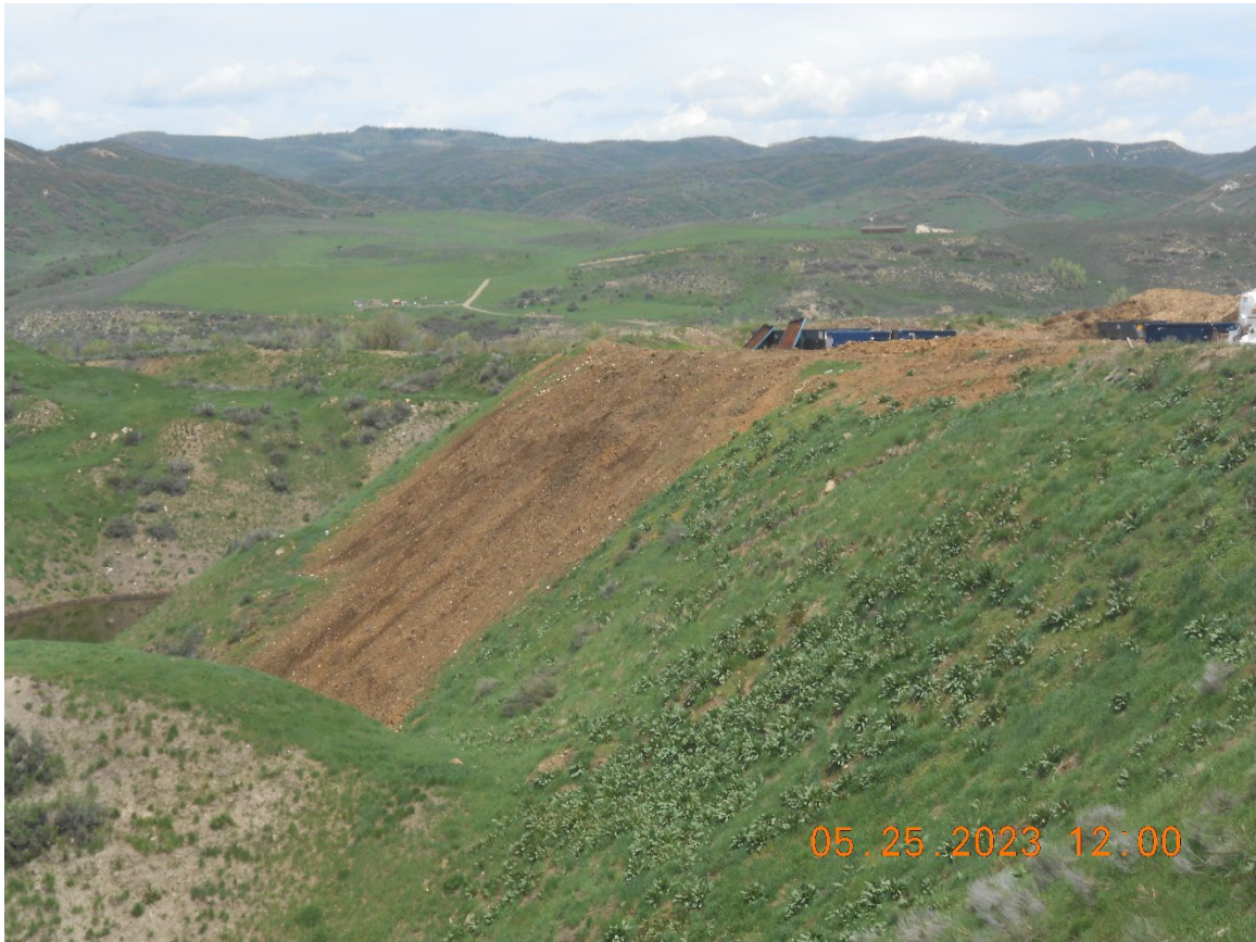
Photo 25: View of western slope at western side of compost pad (note material has been pushed down the slope)
