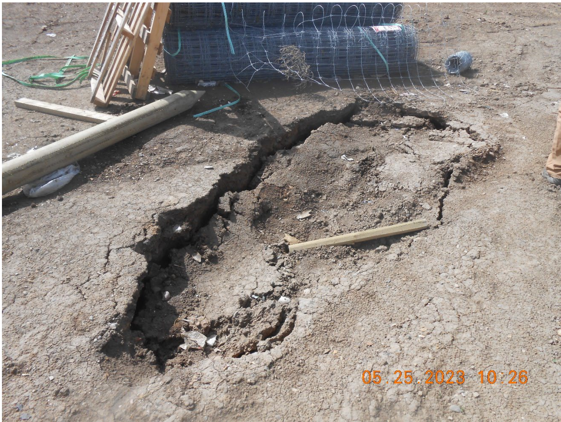
Photo 11: Sunken area attributed to saturated conditions
