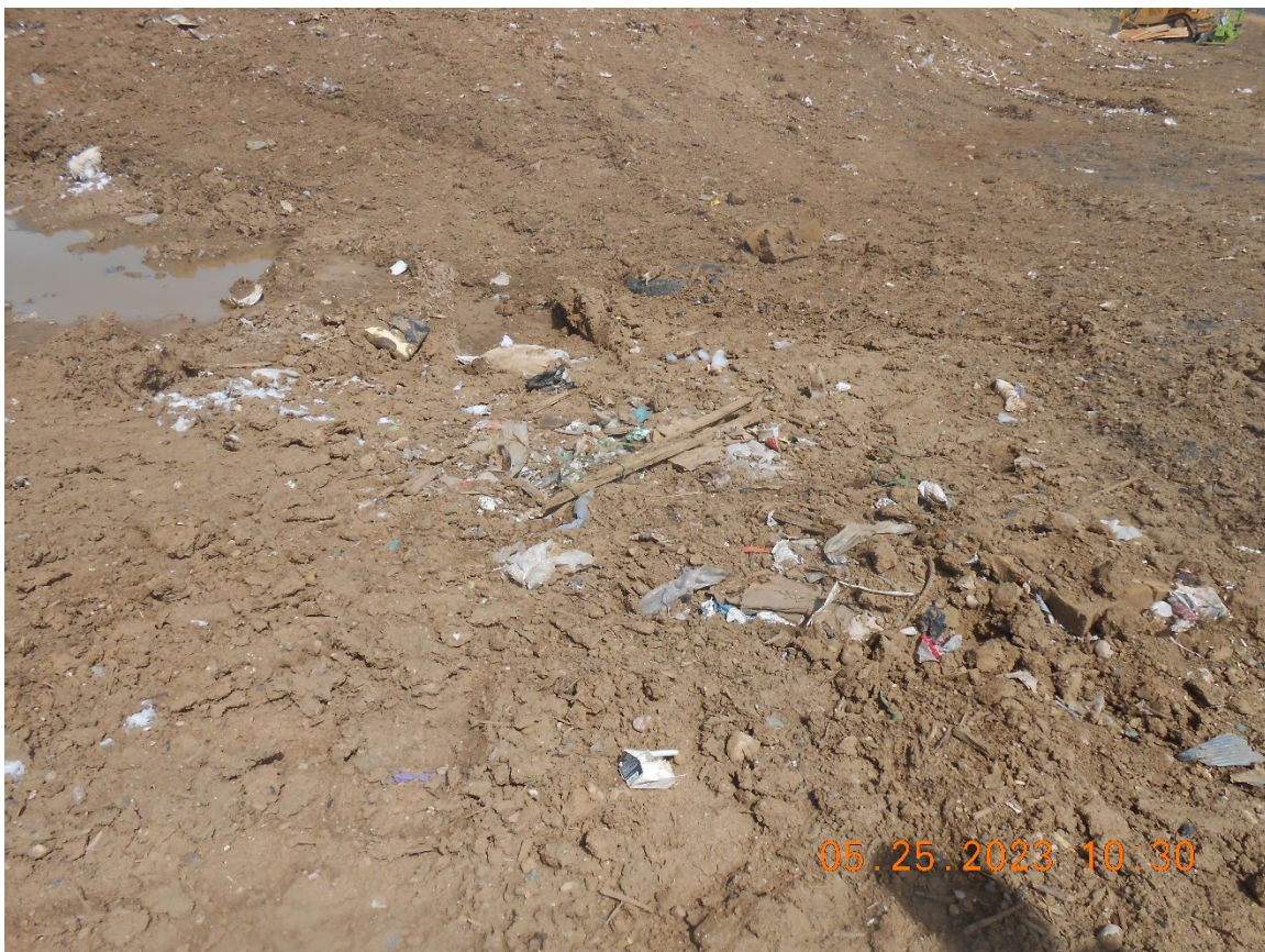
Photo 14: Visible solid waste with insufficient cover south of the working face area
