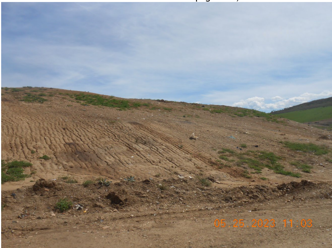
Photo 20: Western slope of landfill (note dark areas indicating seeps)
