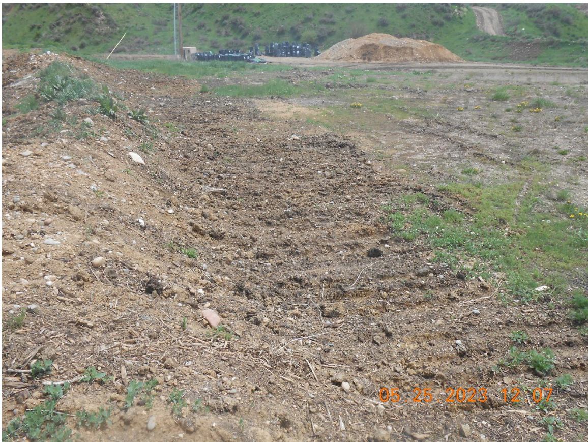
Photo 27: Berm along southern edge of compost pad (note material has been pushed over the berm to the south)
