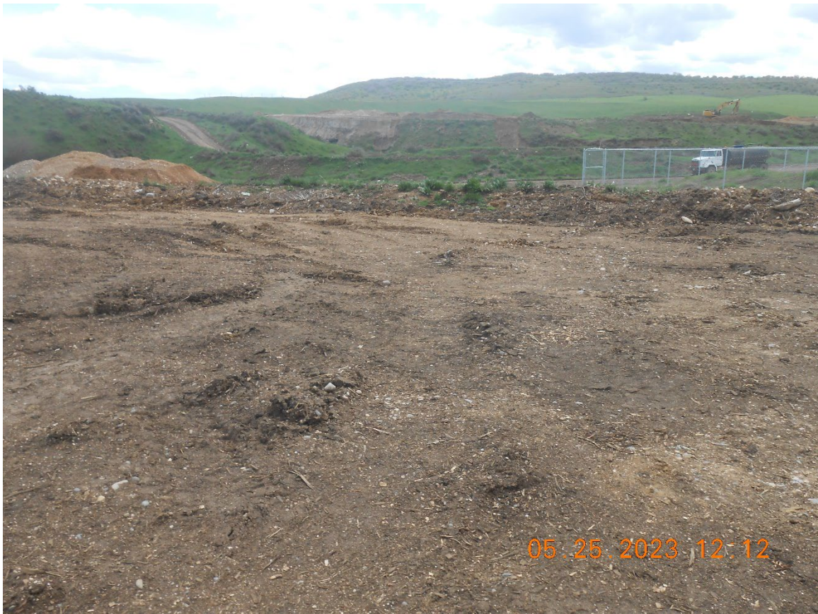
Photo 29: Compost work pad (note grading does not slope north to compost leachate collection pond)
