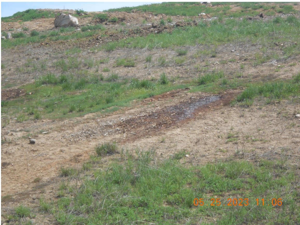
Photo 22: Seep on side slope of landfill (western slope)
