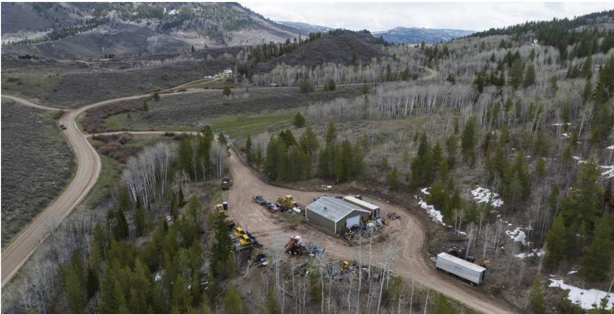
02. Existing maintenance facility on the Stagecoach property.
