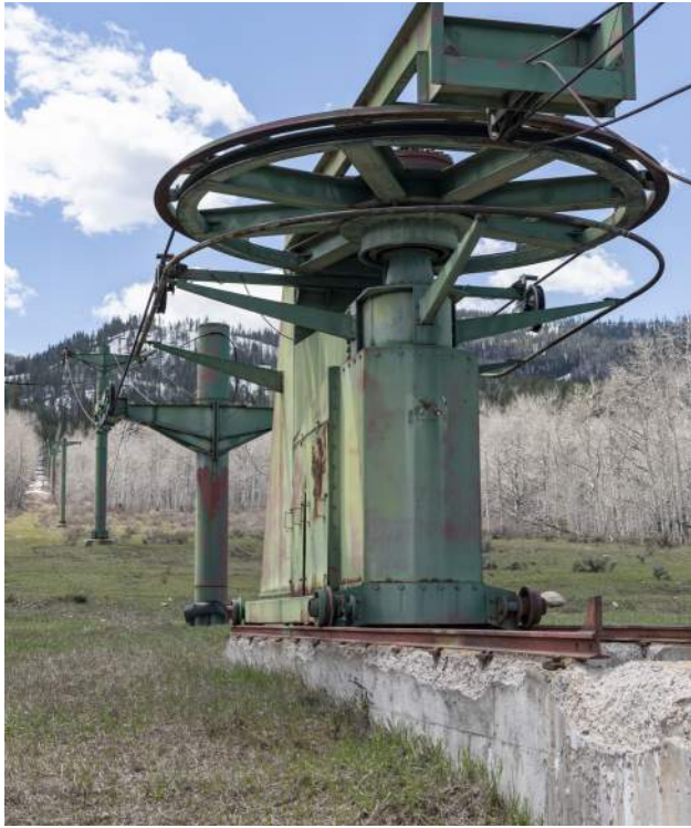
04. Remnants of the existing ski lift on the Stagecoach property.
