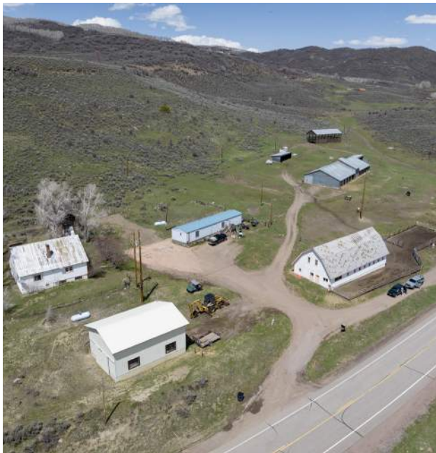
06. Existing facilities located on the Stetson property.
