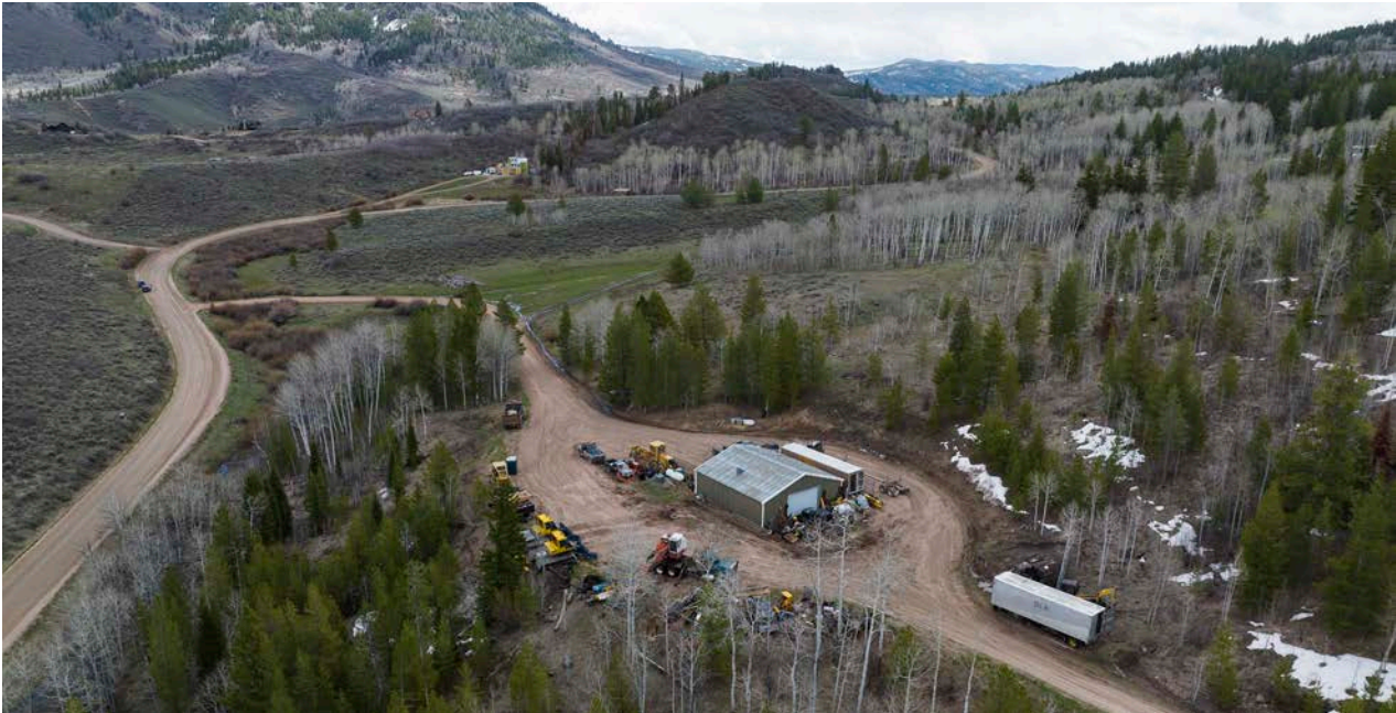
02. Existing maintenance facility on the Stagecoach property.
