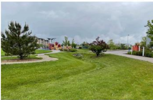
Photograph RPA-3. This grass swale provides treatment of runoff from a parking lot, portions of the building, and sidewalks at a healthcare facility. Photo: WWE.
