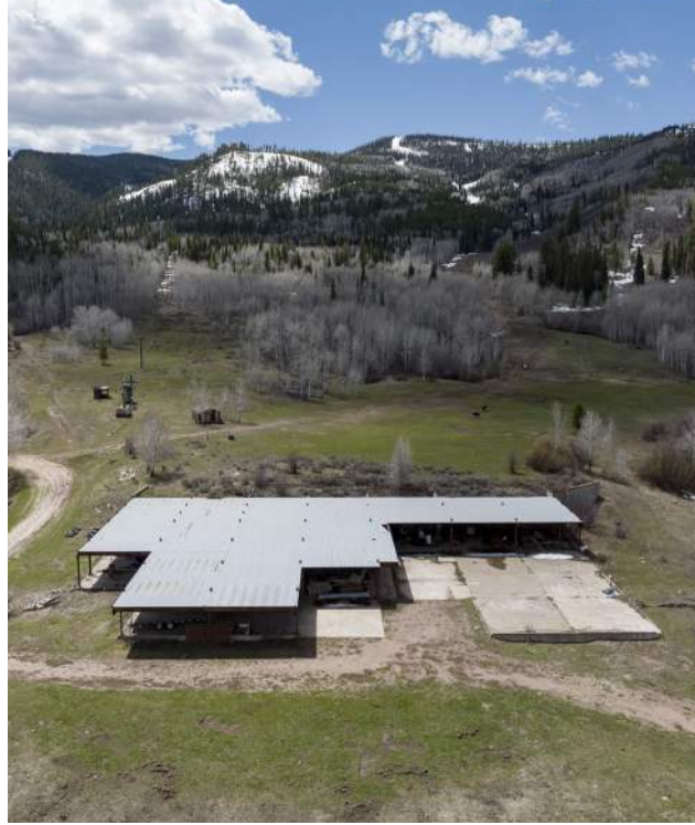
03. Existing structure of the previous base (structure to be removed), looking up to the existing ski runs.
