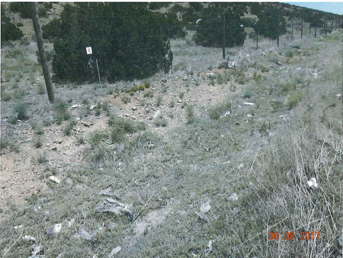
Photo 16: Looking northeast at the stormwater run-on ditch partially covered with gray fly ash.
