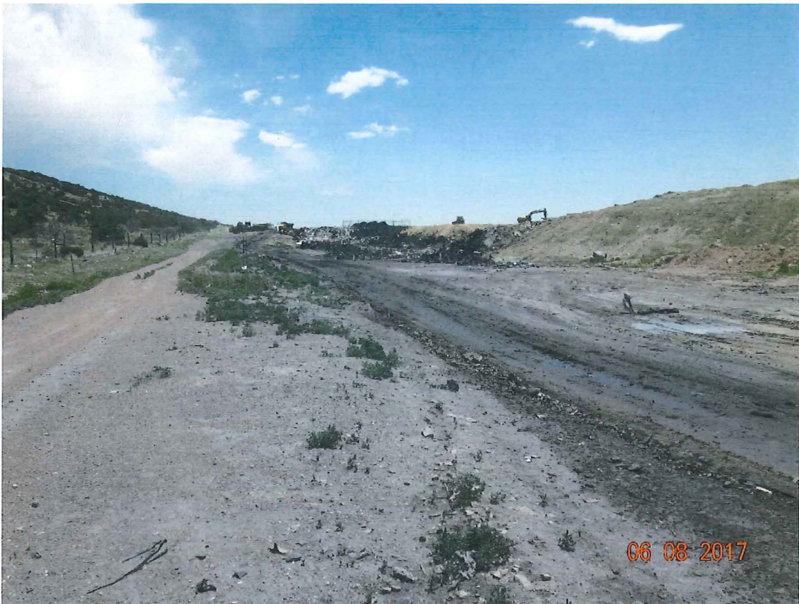
Photo 23: Looking east at the Facility's north boundary road covered with fly ash residue.
