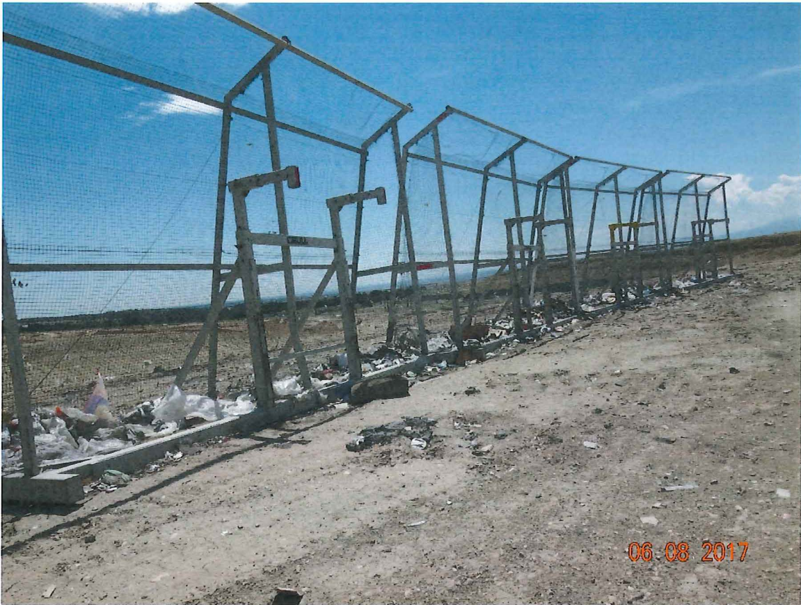
Photo 17: Looking southeast at a movable fence near the waste disposal working face.
