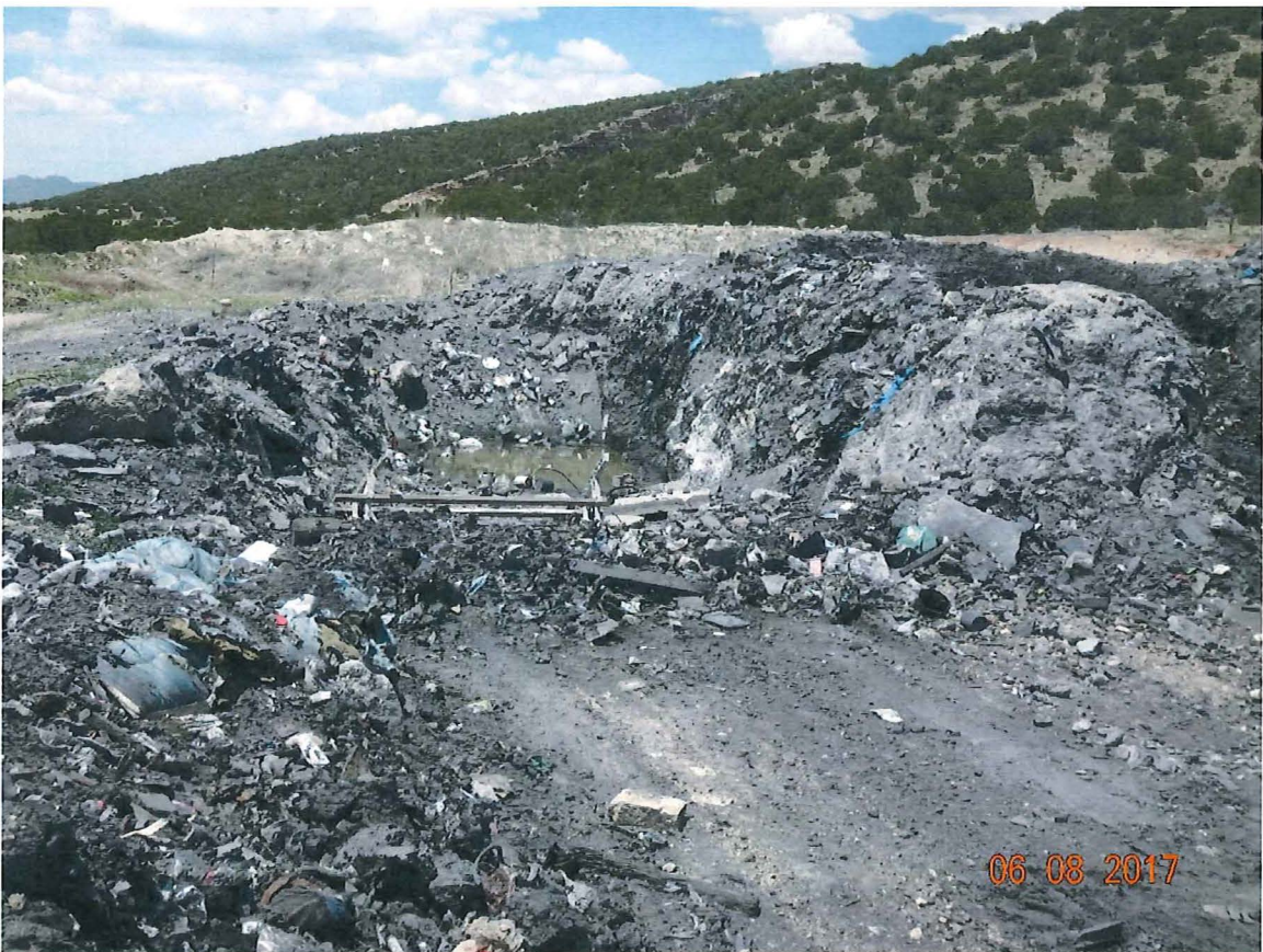
Photo 26: The Facility's southern solidification basin pit and solid waste berms. Looking west.
