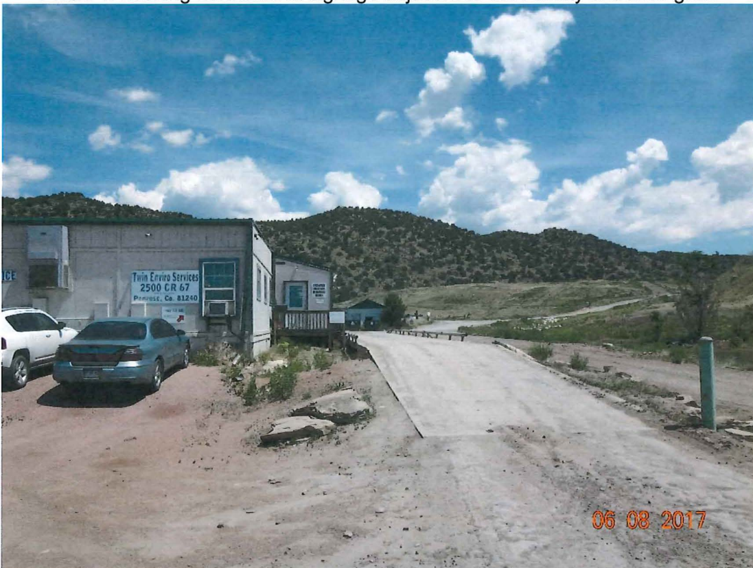
Photo 2: The Facility office and scale at the west portion of the site. Looking northeast.
