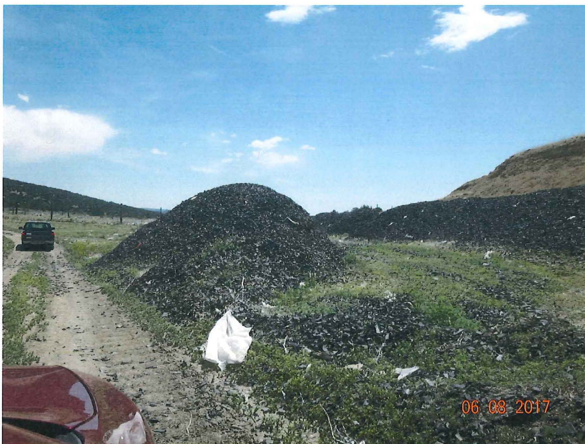
Photo 10: Looking east at stockpiled tire shreds for a leachate drainage layer in the cell under construction.
