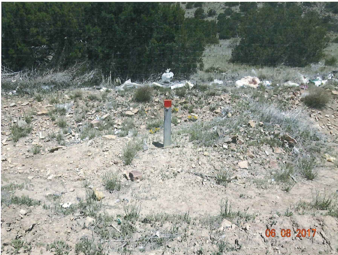
Photo 15: Looking north at a gas monitoring point adjacent to the north boundary fence.
