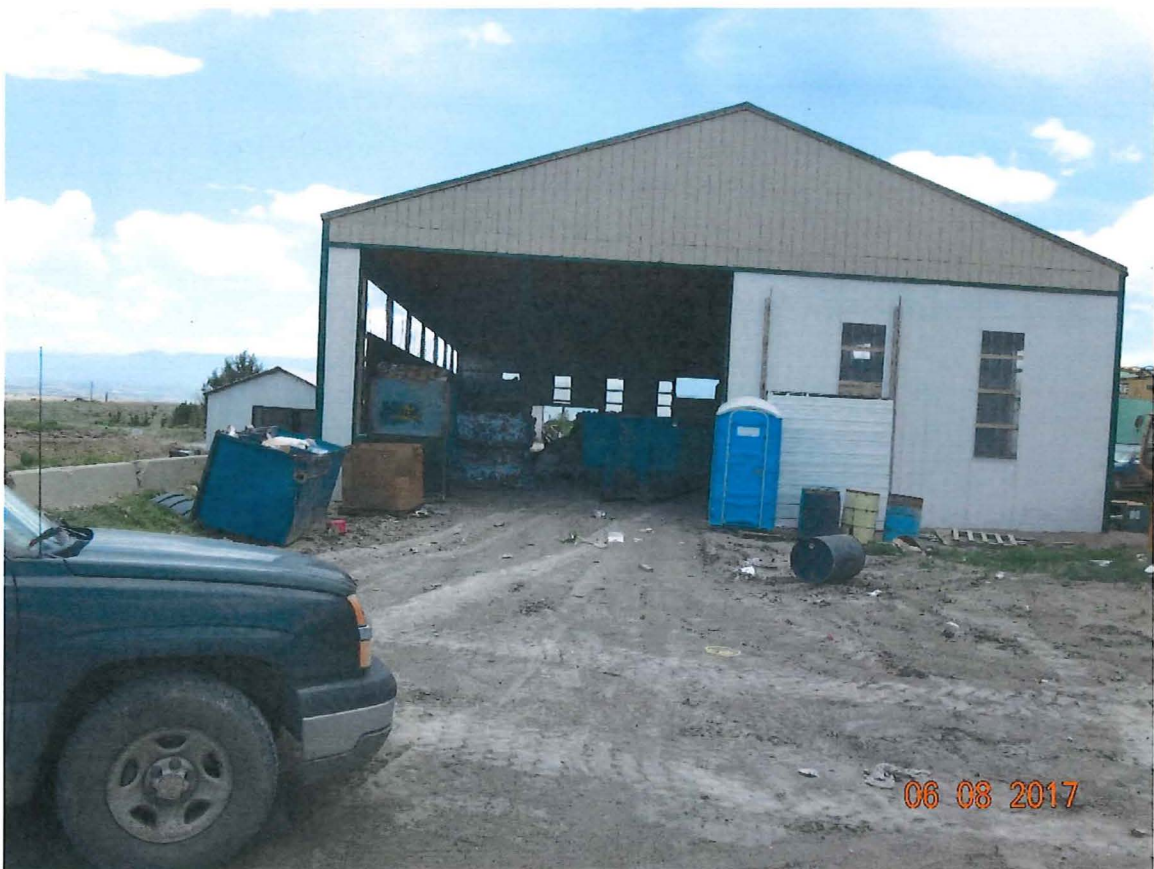
Photo 4: Looking southwest at the recycled materials storage building at the west portion of the Facility.
