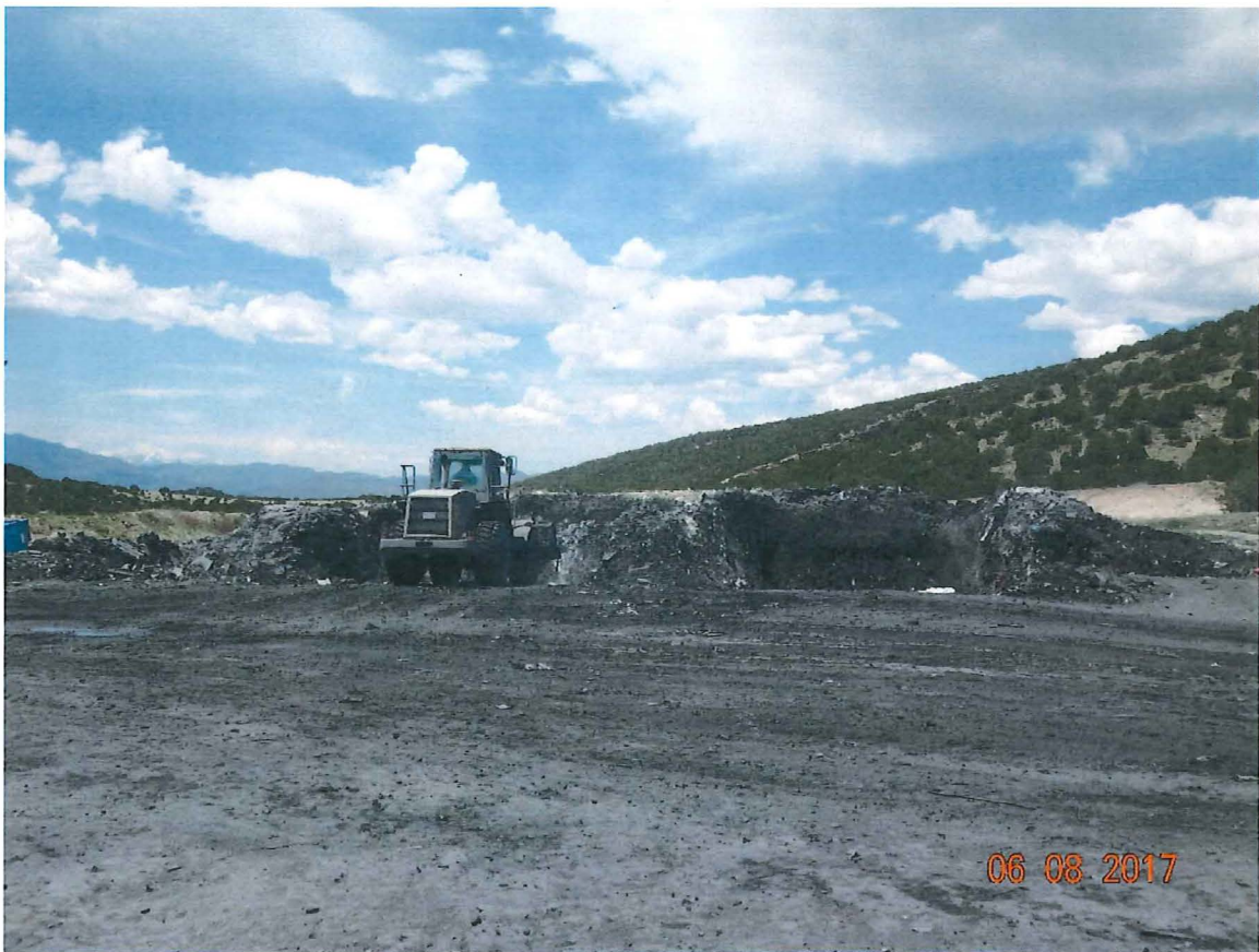
Photo 25: Looking west at the solidification basin pits with berms of fly ash mixed with municipal waste.
