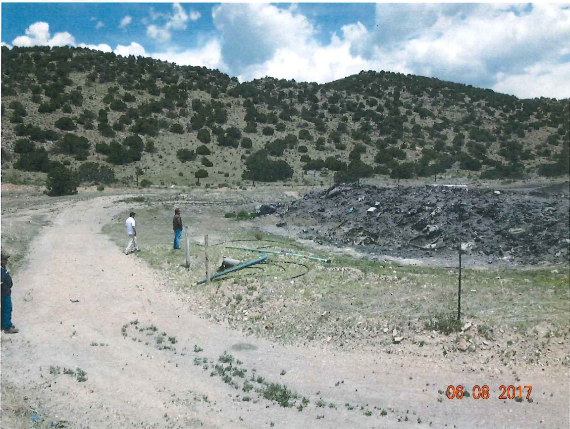
Photo 28: Looking north at the solidification basin leachate removal pipe and uncovered solid waste berms.
