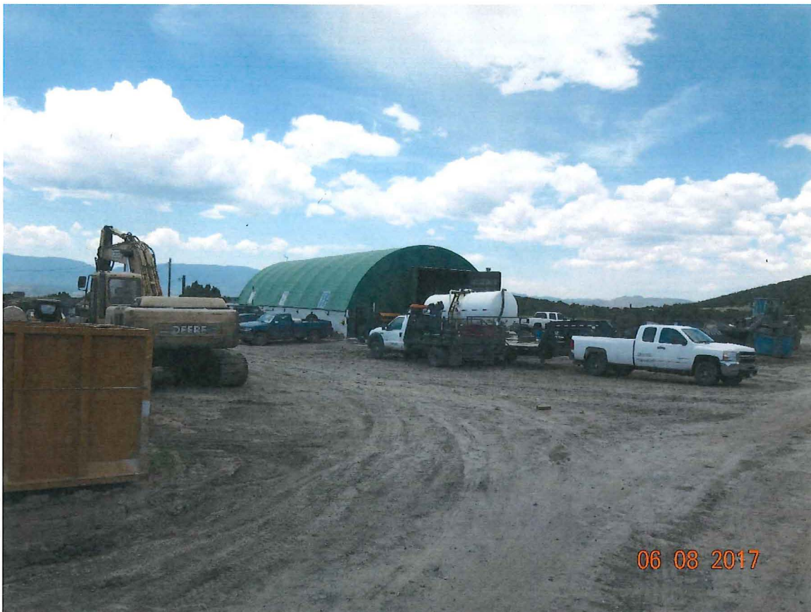
Photo 5: The equipment maintenance building with some Facility equipment. Looking southwest.
