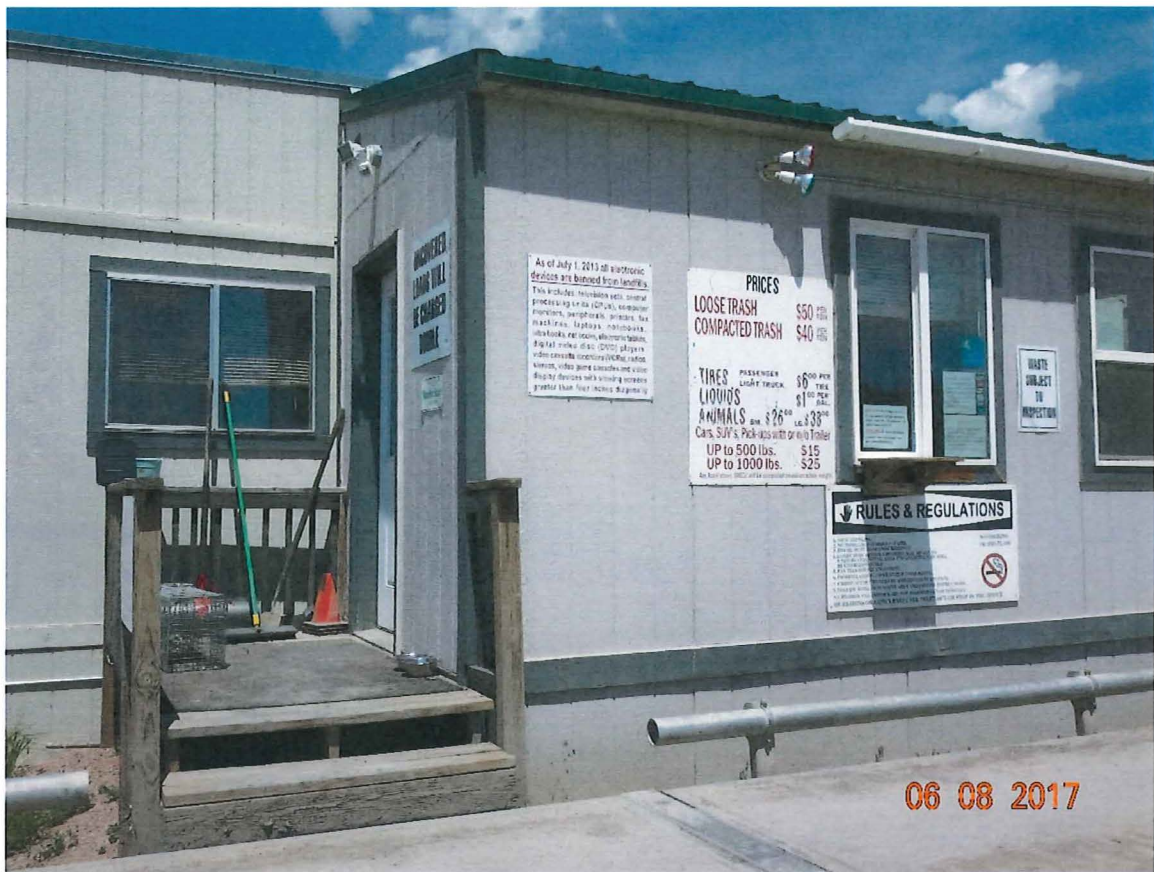
Photo 3: Signs on the Facility office indicating prohibitions, fees, and regulations. Looking north.
