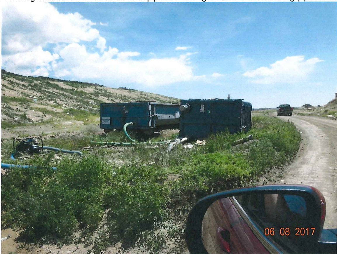
Photo 8: The leachate collection tanks south of the disposal cell. Looking east-northeast.
