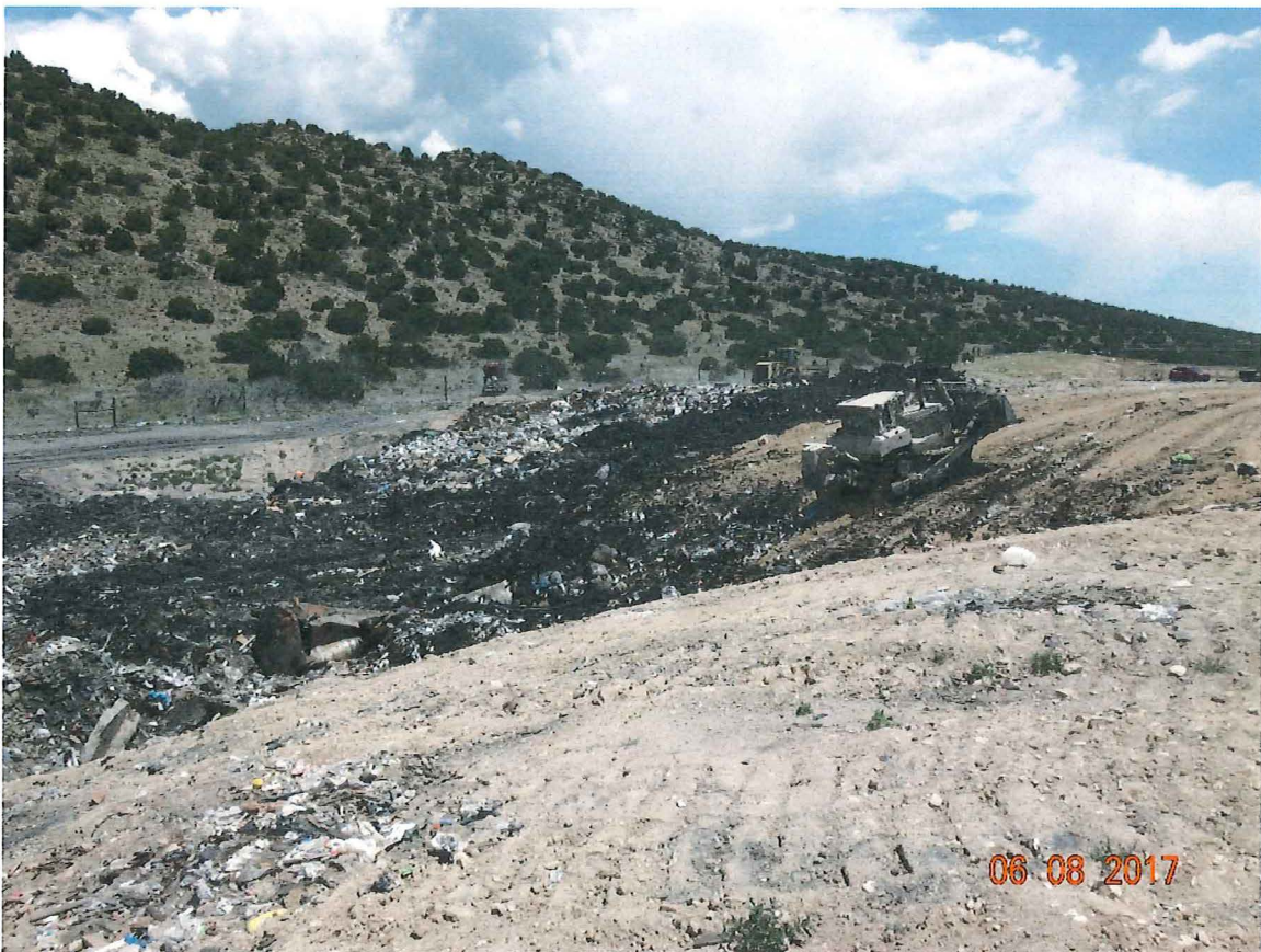
Photo 18: The large working face area at the north-central portion of the Facility. Looking northeast.
