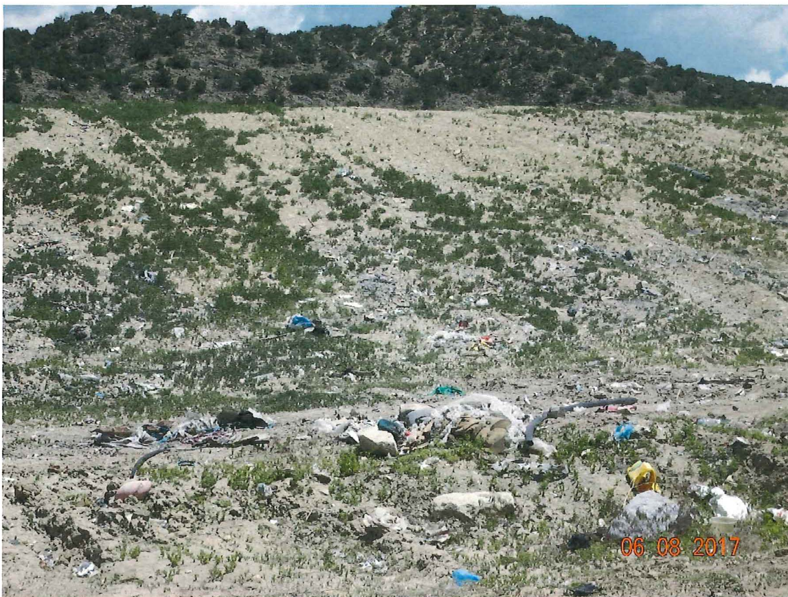
Photo 9: Looking north at the south slope of the disposal cell. Exposed solid waste is visible.
