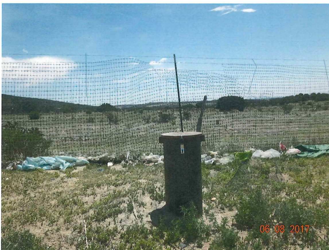
Photo 14: A groundwater monitoring well adjacent to the east boundary fence. Looking east.
