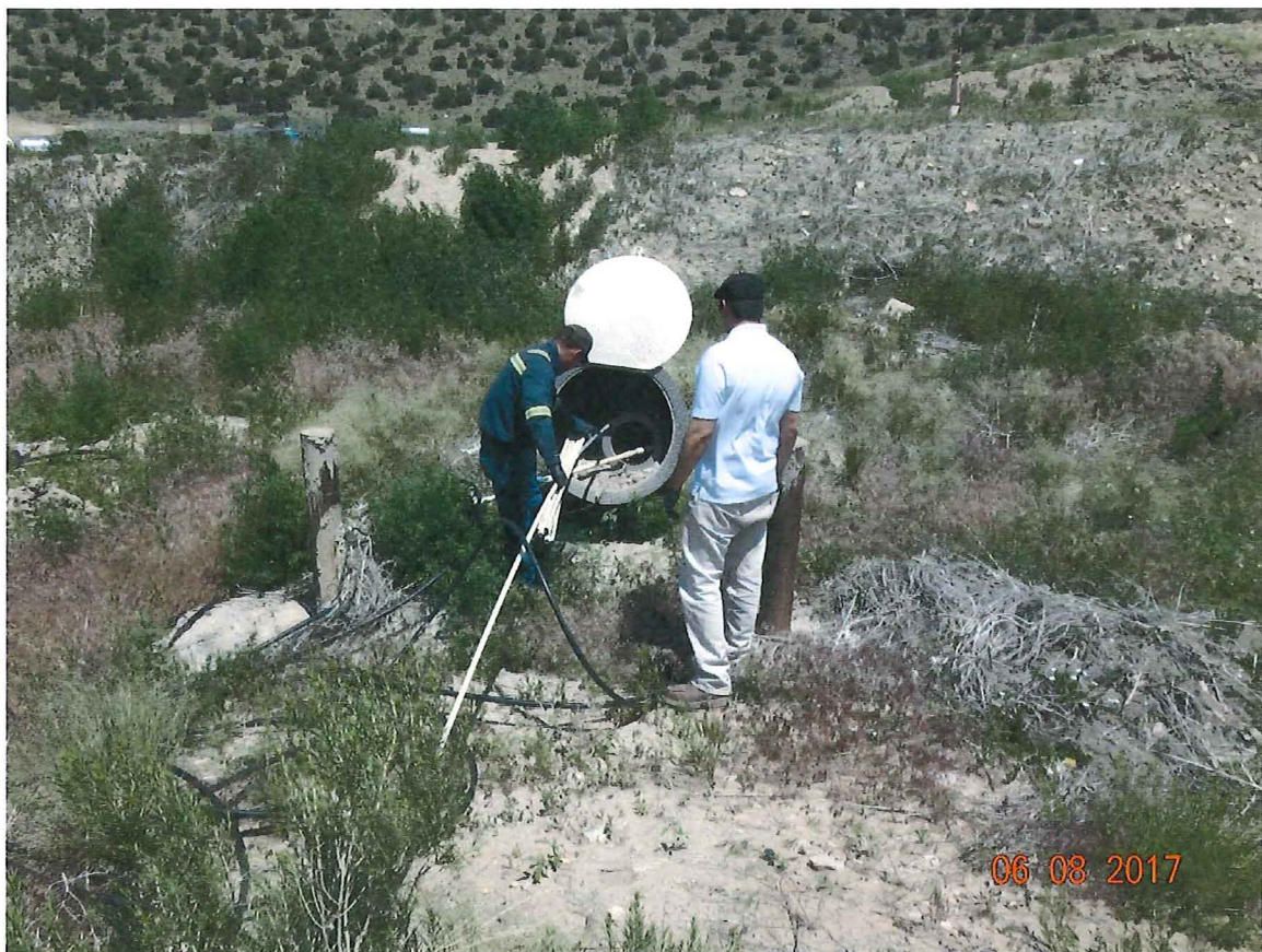
Photo 7: Looking north at the leachate access pipe and casing as the PVC measuring pipe is assembled.
