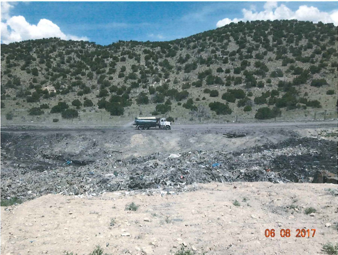
Photo 20: Water being applied north of the combined working face and fly ash removal area. Looking north.
