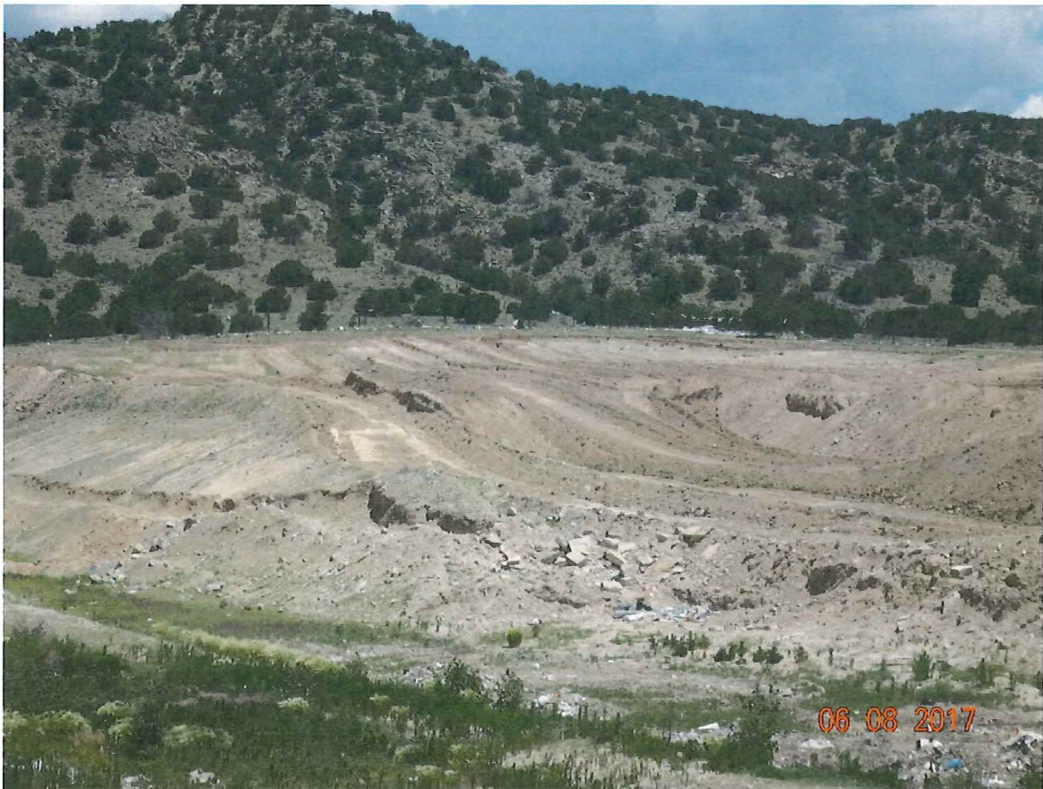
Photo 11: Looking northeast at the cell construction area at the east portion of the Facility.
