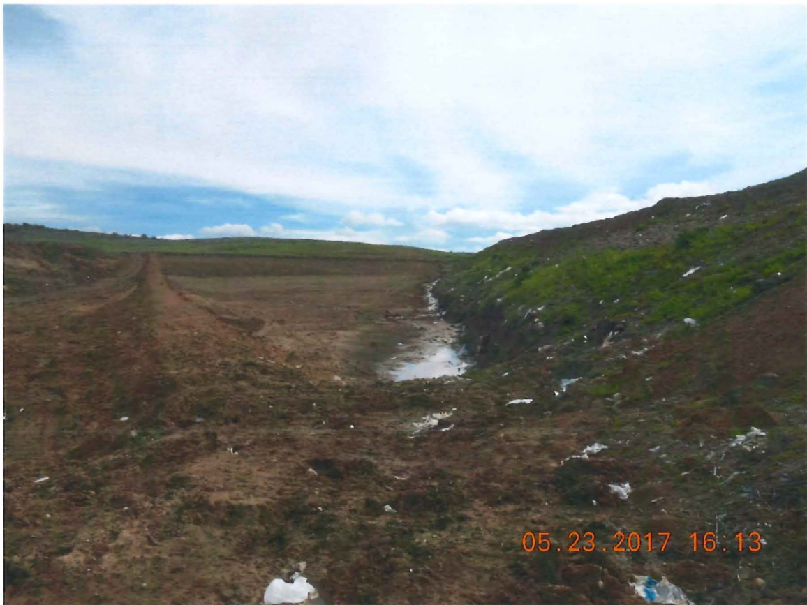
Photo 39: Exposed waste (insufficient cover) in MOD 6A/7A area
