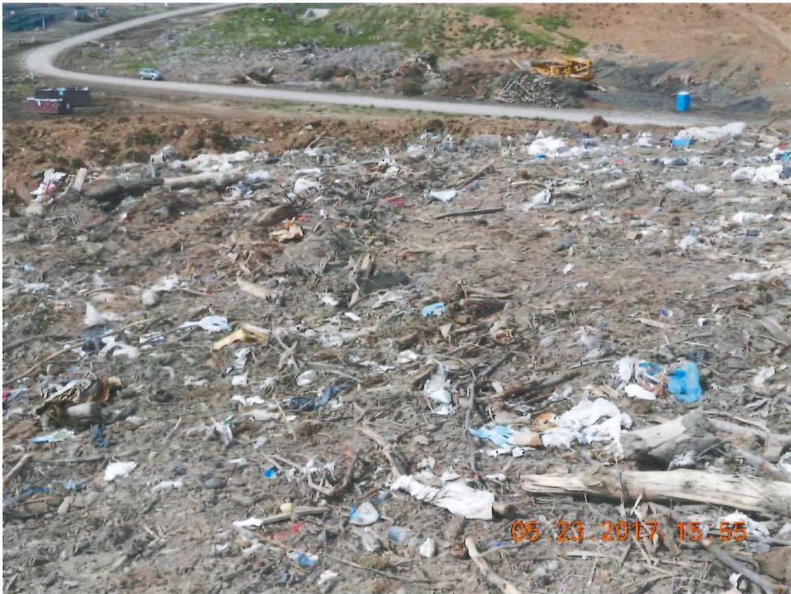
Photo 31: Exposed waste (insufficient cover) near working face
