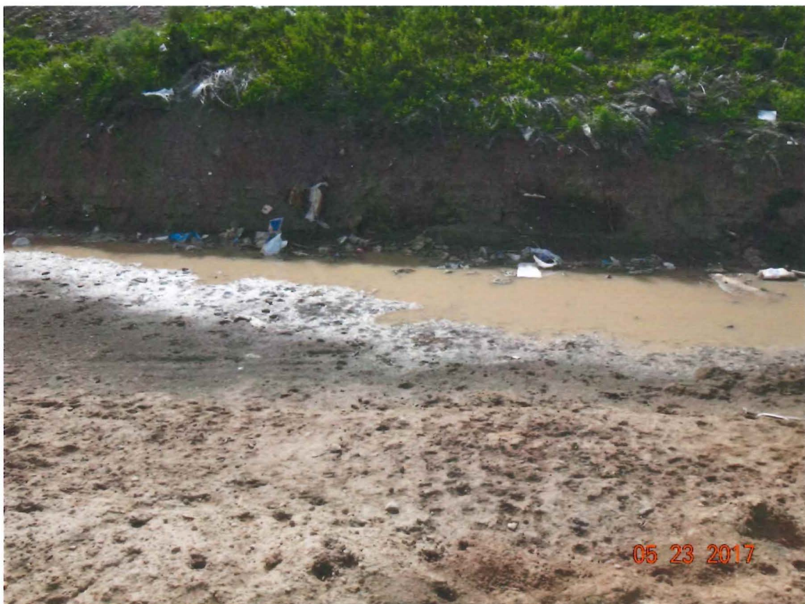
Photo 40: Exposed waste (insufficient cover) in MOD 6A/7A area
