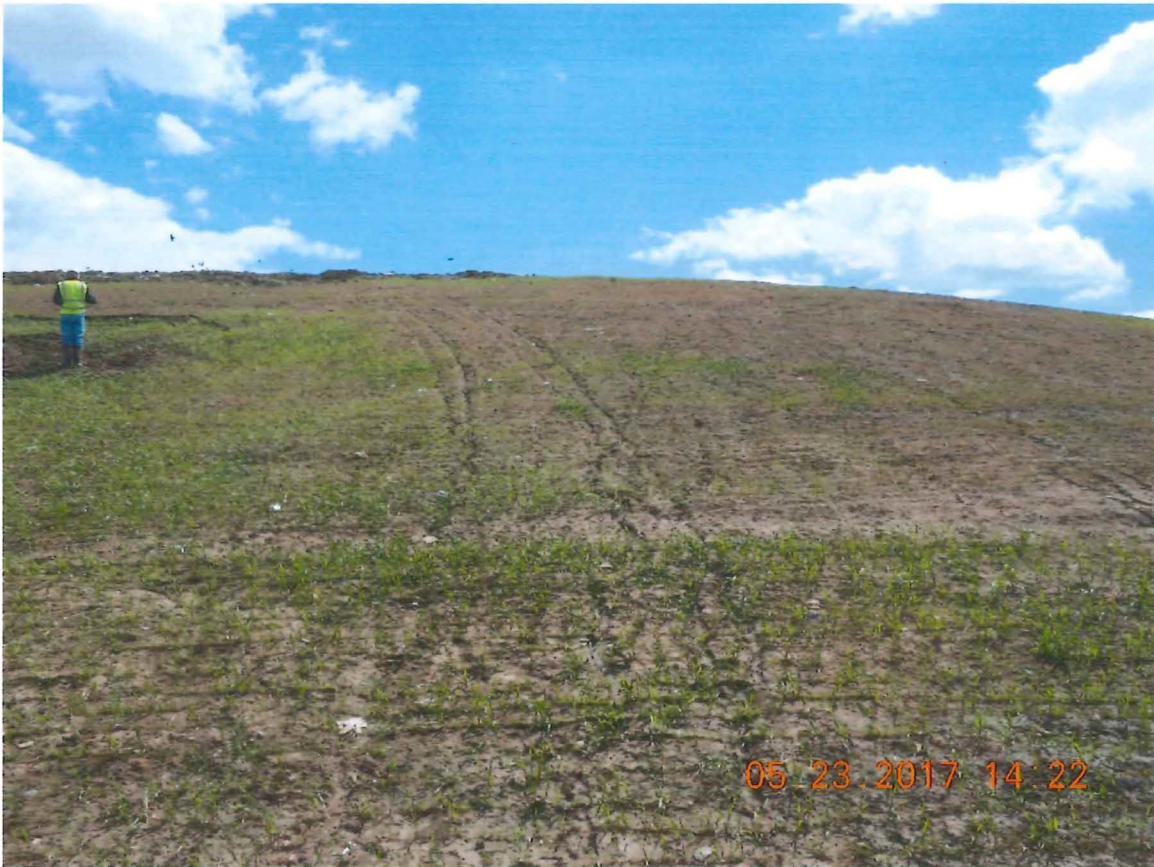
Photo 35: Erosion rilling on western slope of active fill area
