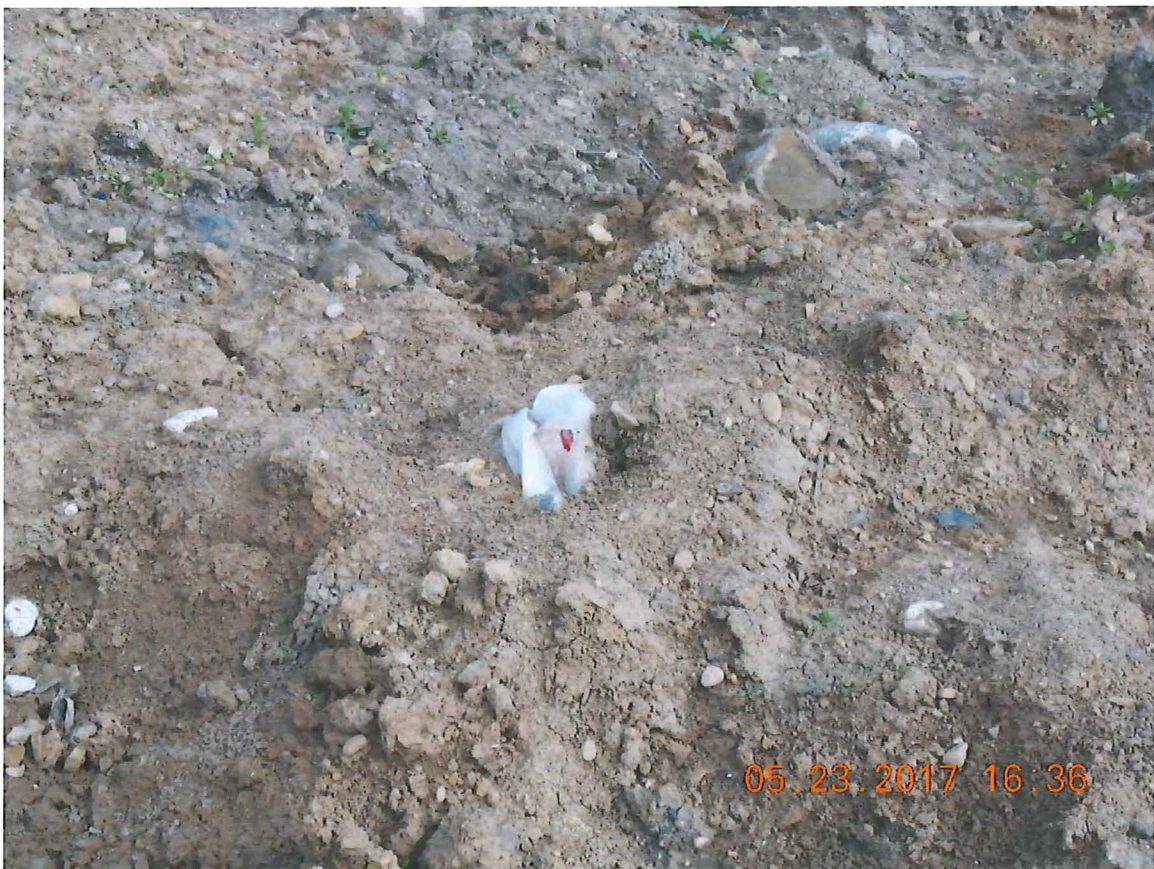
Photo 46: Uncovered asbestos waste
