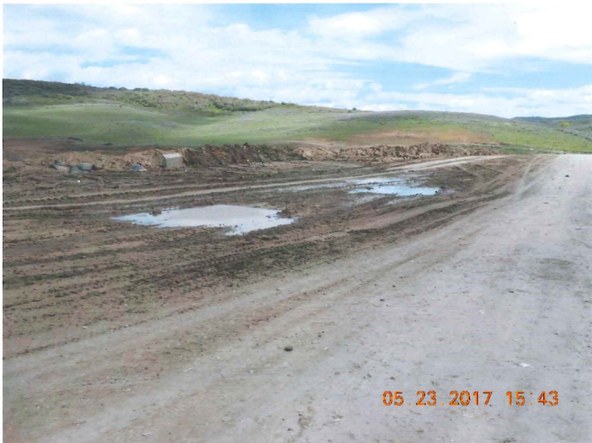
Photo 28: Ponding of water near working face
