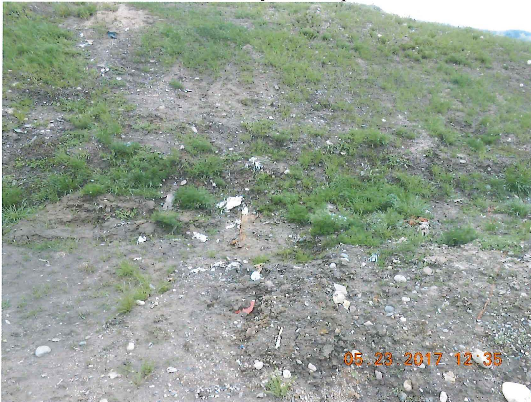
Photo 1: Exposed waste in hillside next to new Material Recovery Facility (MRF)
