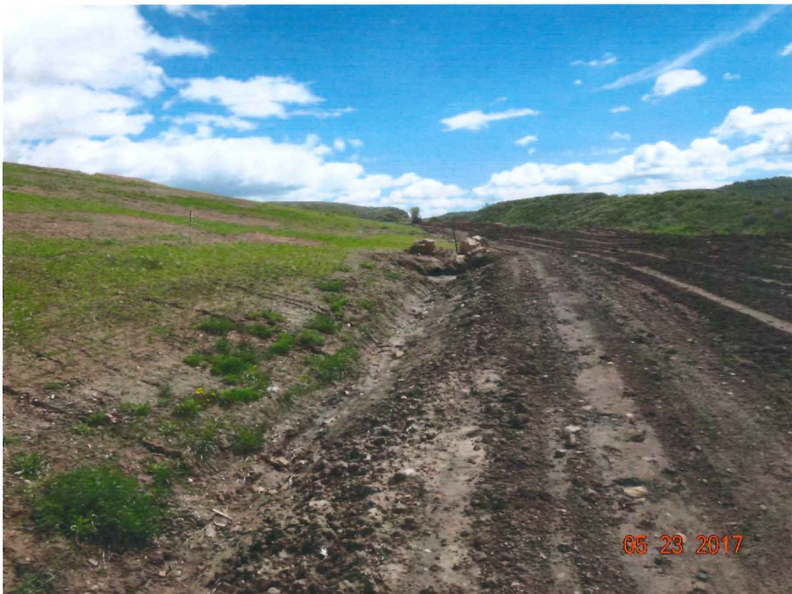
Photo 24: Storm water ditch along W slope of active fill area (also note culvert in background which may be removed)
