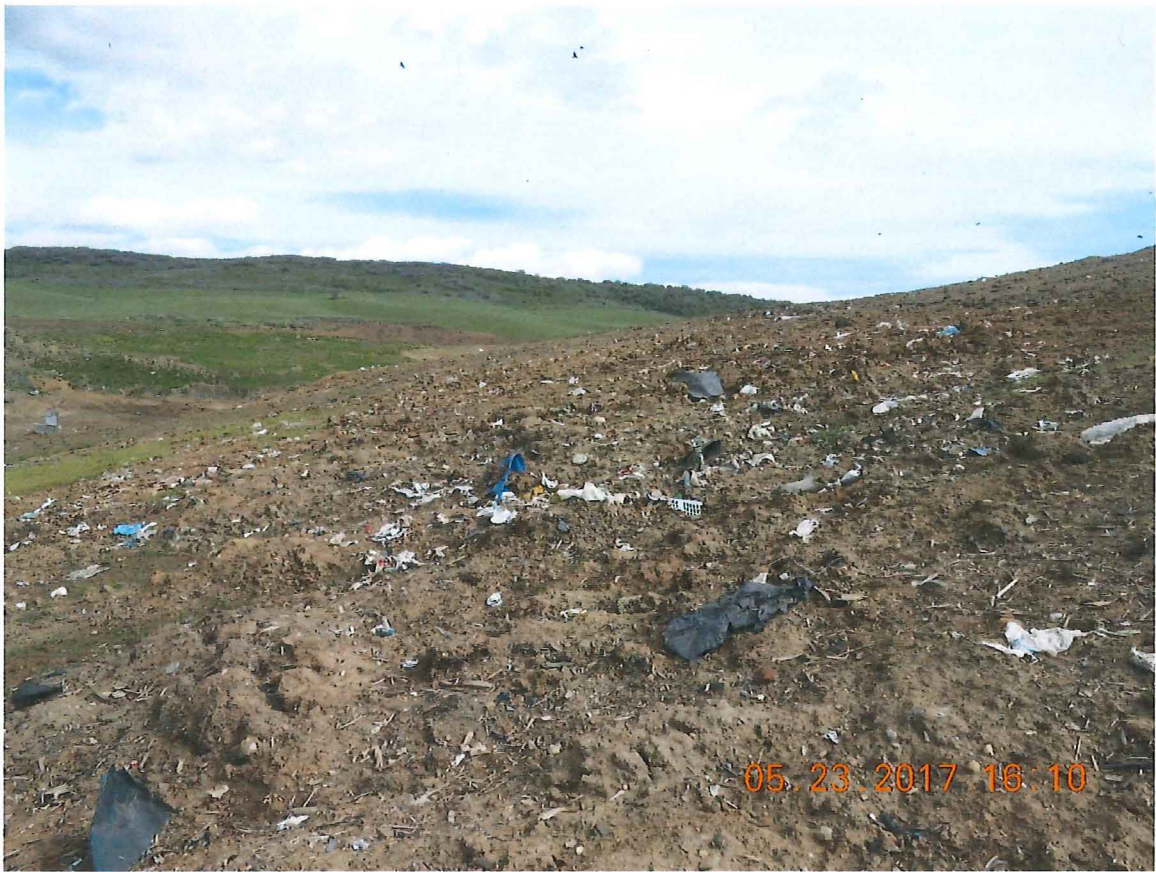
Photo 33: Exposed waste (insufficient cover) on northern slope of active fill area
