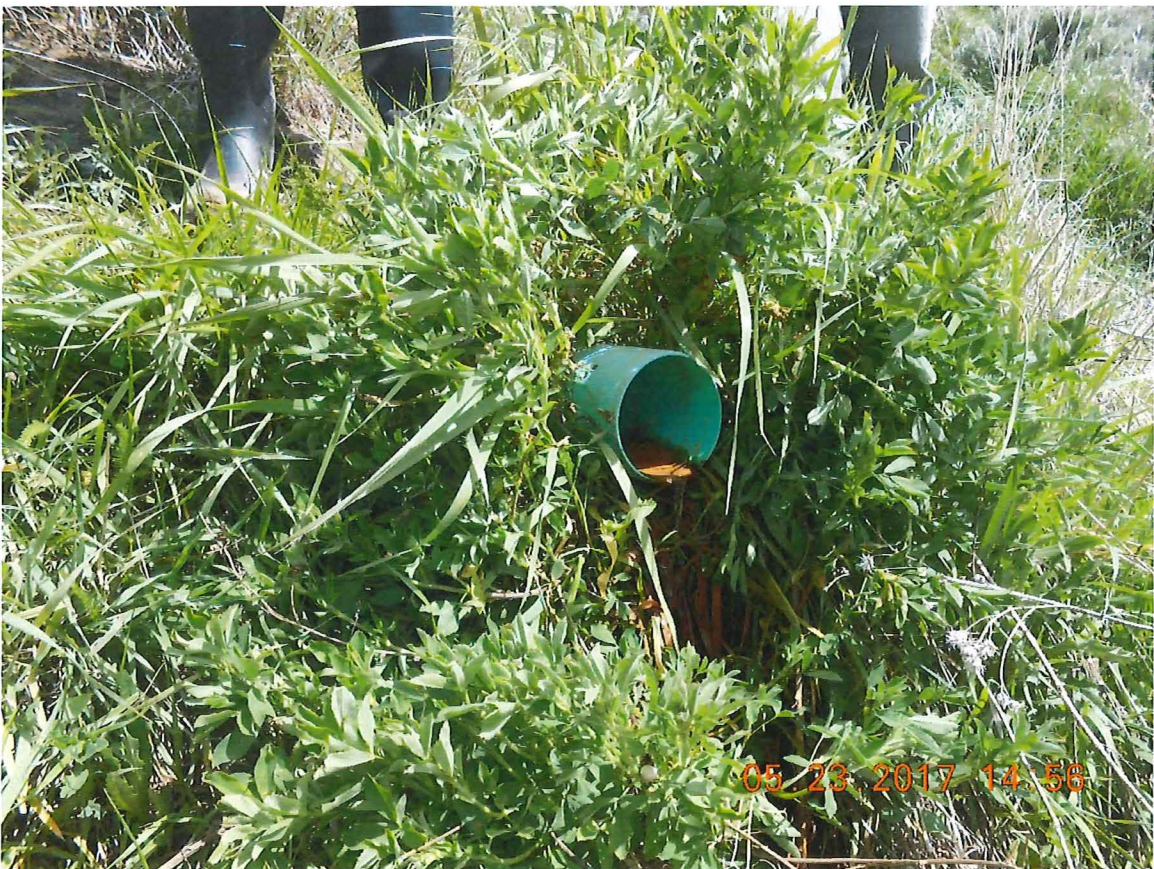
Photo 26: Original underdrain discharge point
