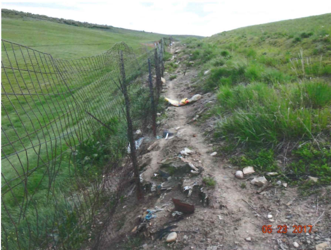
Photo 43: Exposed waste (insufficient cover) in Pit 6 area
