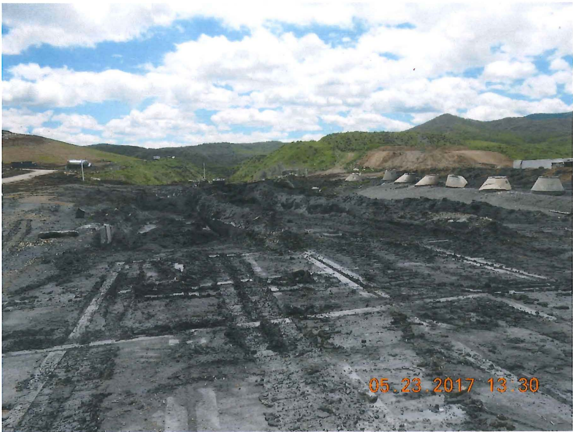
Photo 17: Ash all over ground surface around solidification basin
