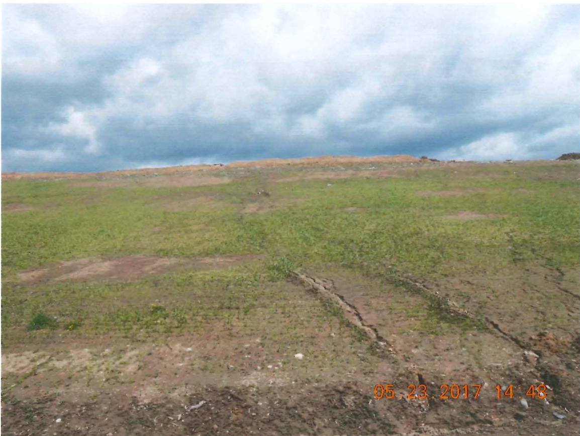
Photo 36: Erosion rilling on western slope of active fill area
