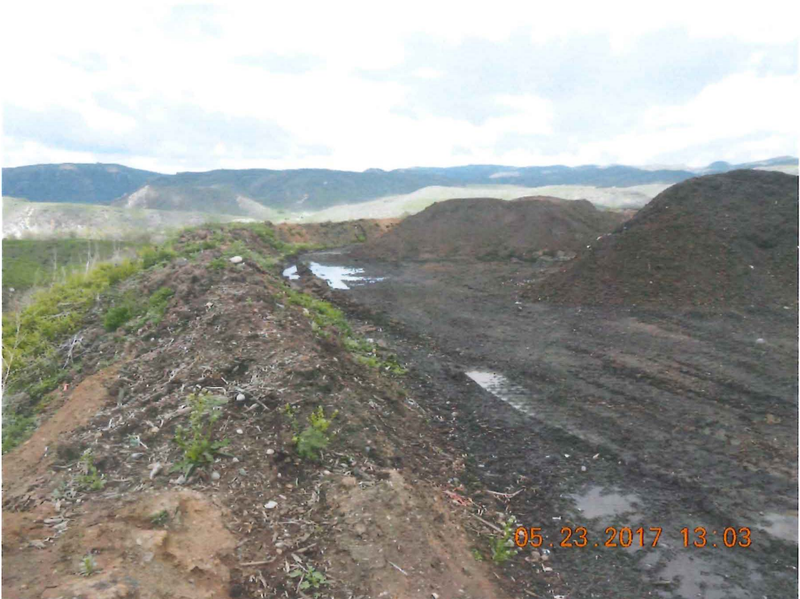
Photo 8: Newly enhanced berms around compost storage area
