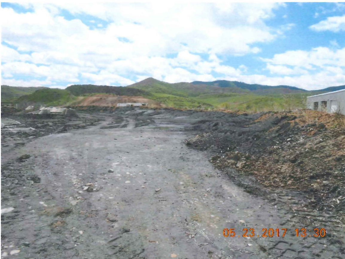
Photo 16: Ash all over ground surface around solidification basin
