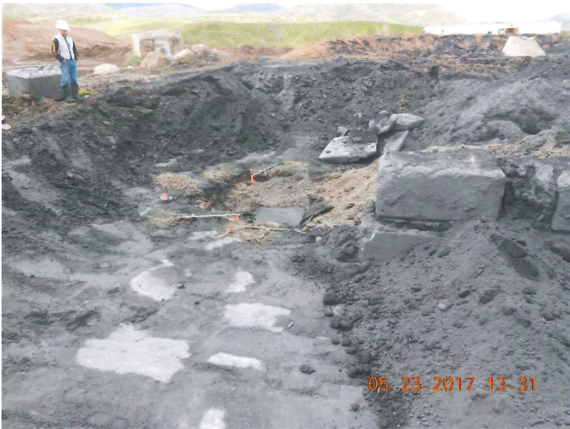
Photo 19: Excavation to expose coupon in the solidification basin
