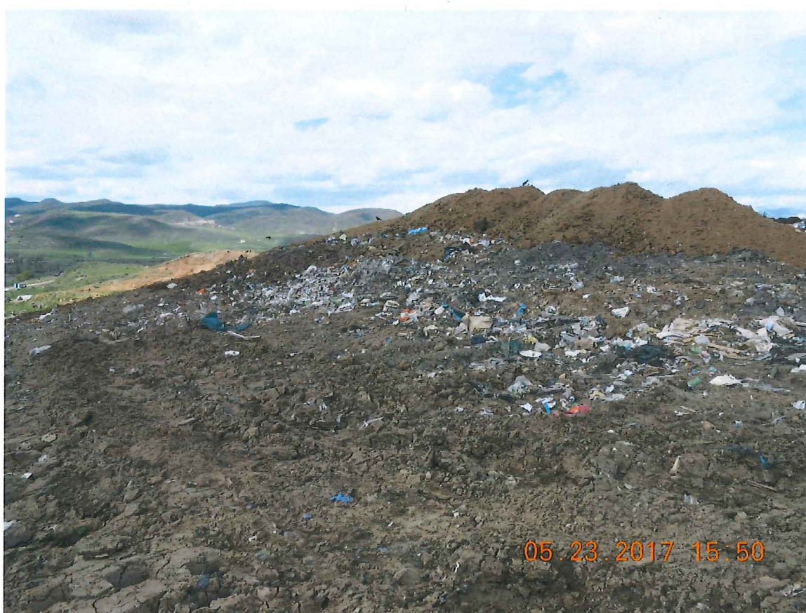
Photo 30: Exposed waste (insufficient cover) near working face
