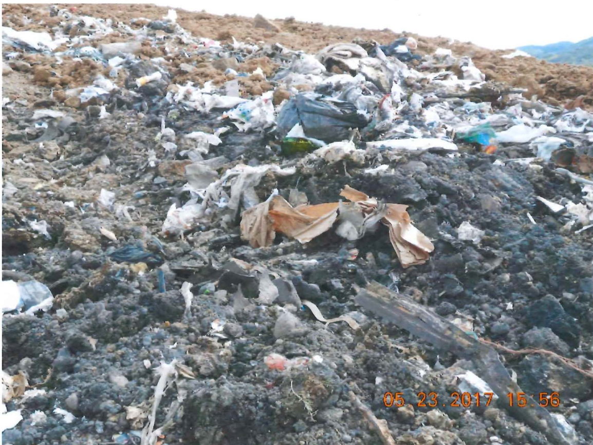
Photo32: Exposed waste (insufficient cover) near working face
