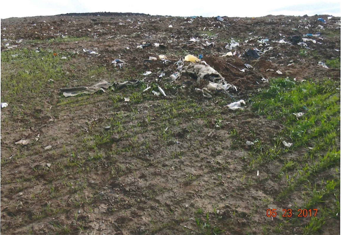
Photo 34: Exposed waste (insufficient cover) on northern slope of active fill area
