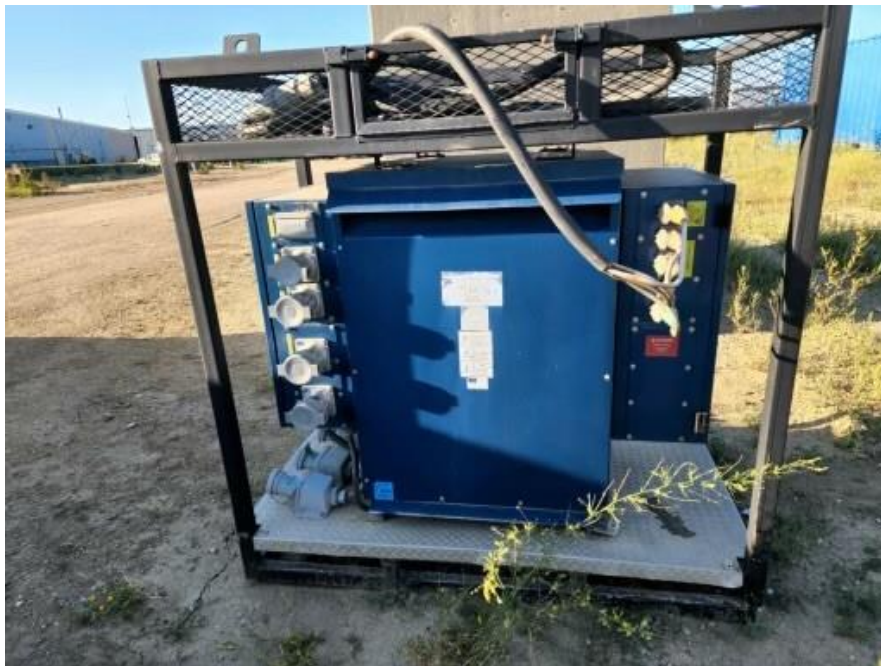
Figure 4: 480V/220V 112KVA Transformer
