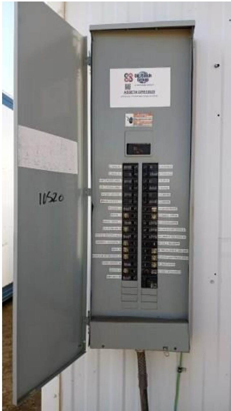
Figure 9: THU 100 amp service breaker panels
